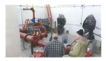
Pumps and motors are in place. Piping is now completed. Items are being covered or masked in preparation for the painters.
