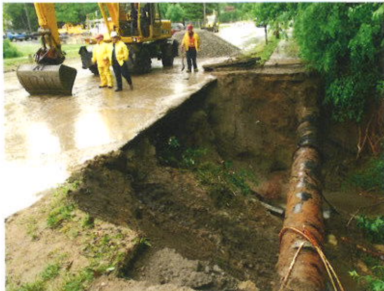
Figure 22. Fixing water main breaks is the most common direct conservation effort undertaken by Minnesota water suppliers.
