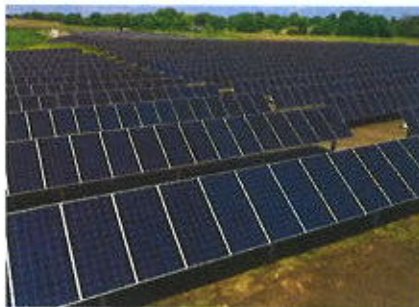
BUFFALO SOLAR BUFFALO TOWNSHIP, MN 7 MW, SOLAR
