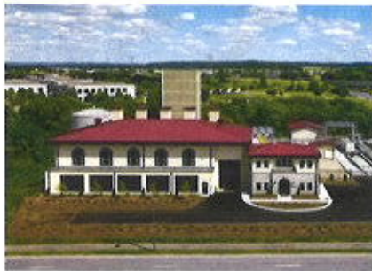
SHAKOPEE ENERGY PARK SHAKOPEE, MN 46 MW, NATURAL GAS
