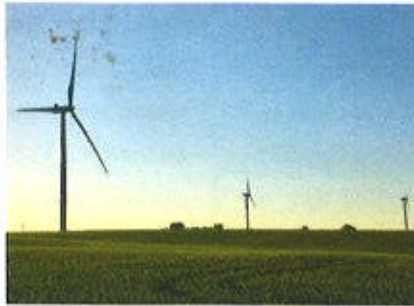
BLACK OAK GETTY WIND FARM STEARNS COUNTY, MN 78 MW, WIND
