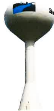
2065 Dominion 500 K - 2002 TANK 4 (896')
