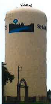
870 10 th Ave 2 MG - 1966 TANK 1 (818')
