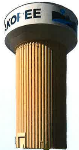
803 Canterbury Rd 1.5 MG - 1980 TANK3 (770')
