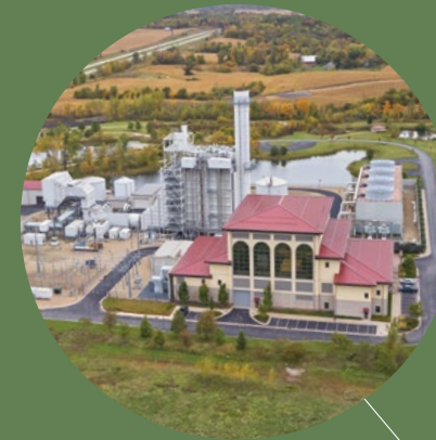
FARIBAULT ENERGY PARK FARIBAULT, MN 300 MW, Natural Gas
