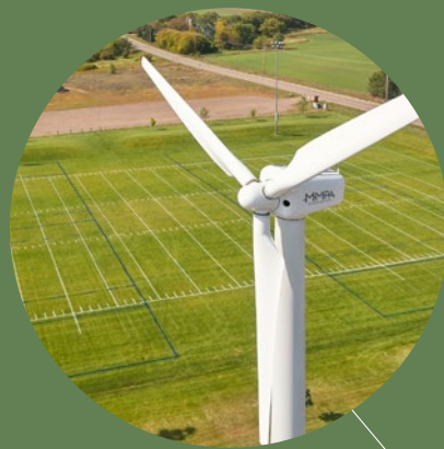
HOMETOWN WINDPOWER MMPA COMMUNITIES 1.9 MW, Wind
