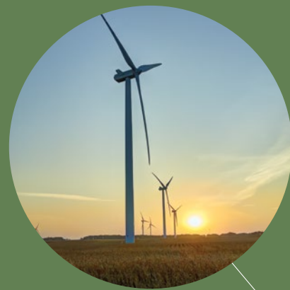
OAK GLEN WIND FARM STEELE COUNTY, MN 44 MW, Wind
