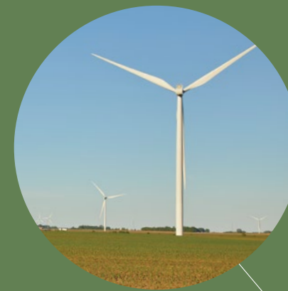
BLACK OAK GETTY WIND FARM STEARNS COUNTY, MN 78 MW, Wind
