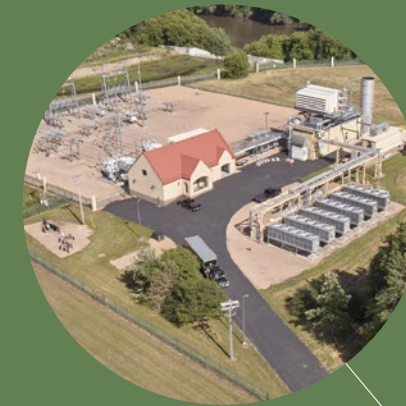
MINNESOTA RIVER STATION CHASKA, MN 49 MW, Natural Gas
