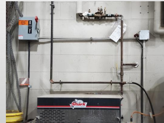
Isolation Backflow Assembly
