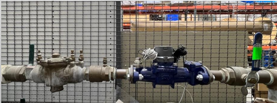
Containment Backflow Assembly
