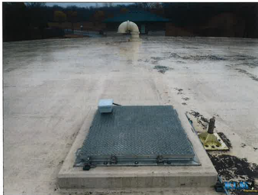
Photo No. 12 Bilco access hatch
