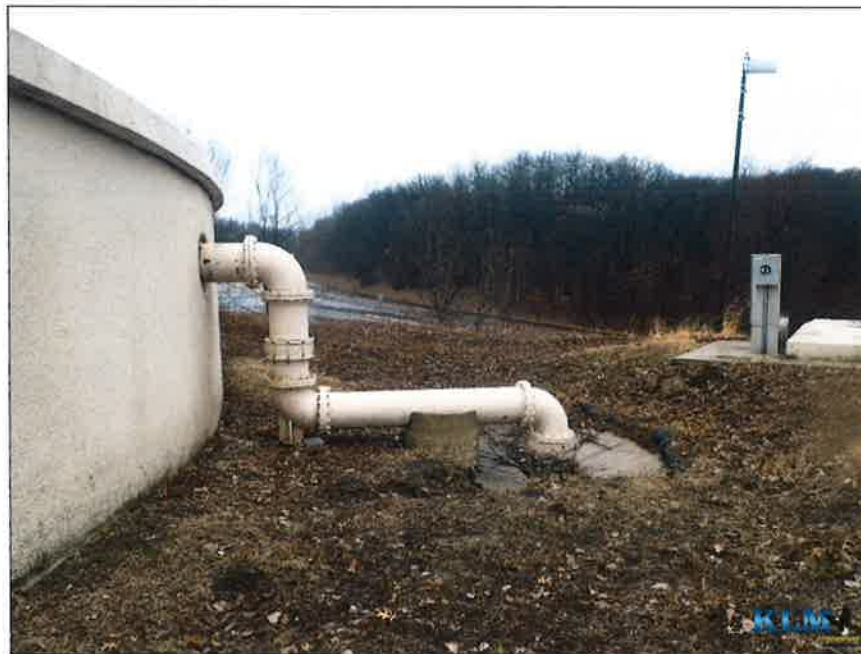
Photo No. 16 Overflow pipe and catch basin
