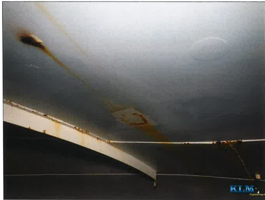
Photo No. 5 Condition of roof stiffener and plates
