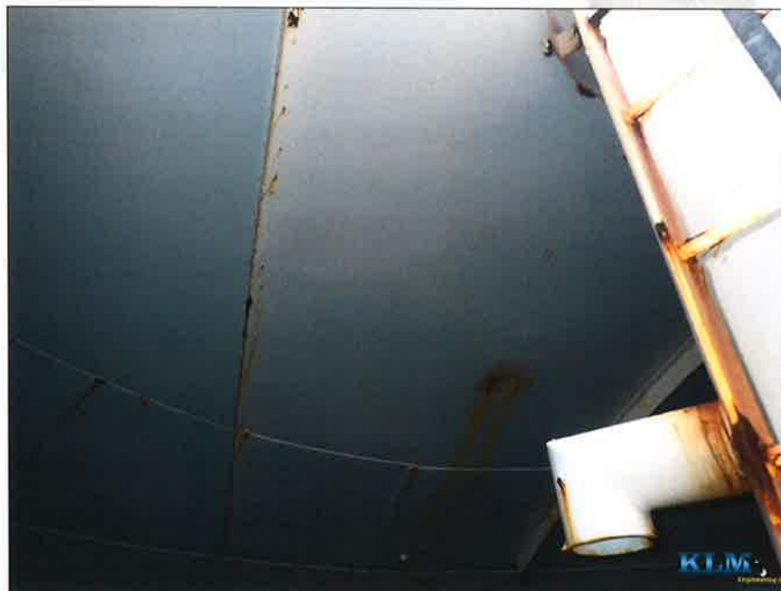
Photo No. 4 Condition of roof stiffeners and plates Overflow pipe inlet visible
