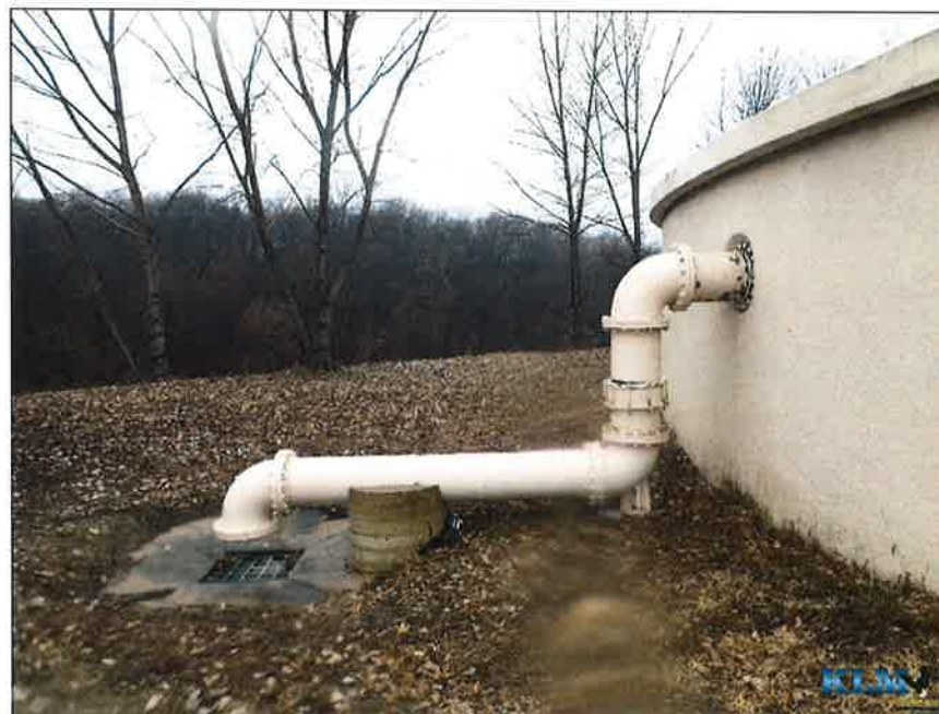
Photo No. 16 Overflow pipe and catch basin
