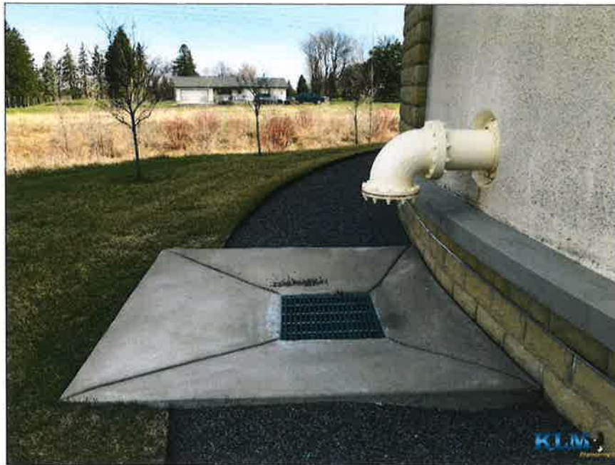
Photo No. 23 Overflow pipe discharge and catch basin
