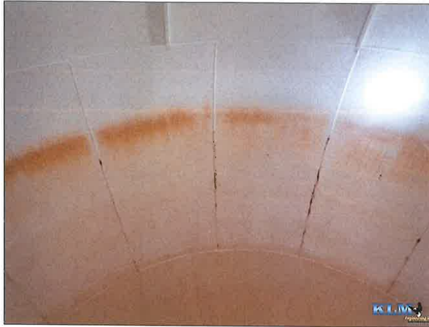
Photo No. 7 View of shell Staining visible with pinhole coating failures on weld seams
