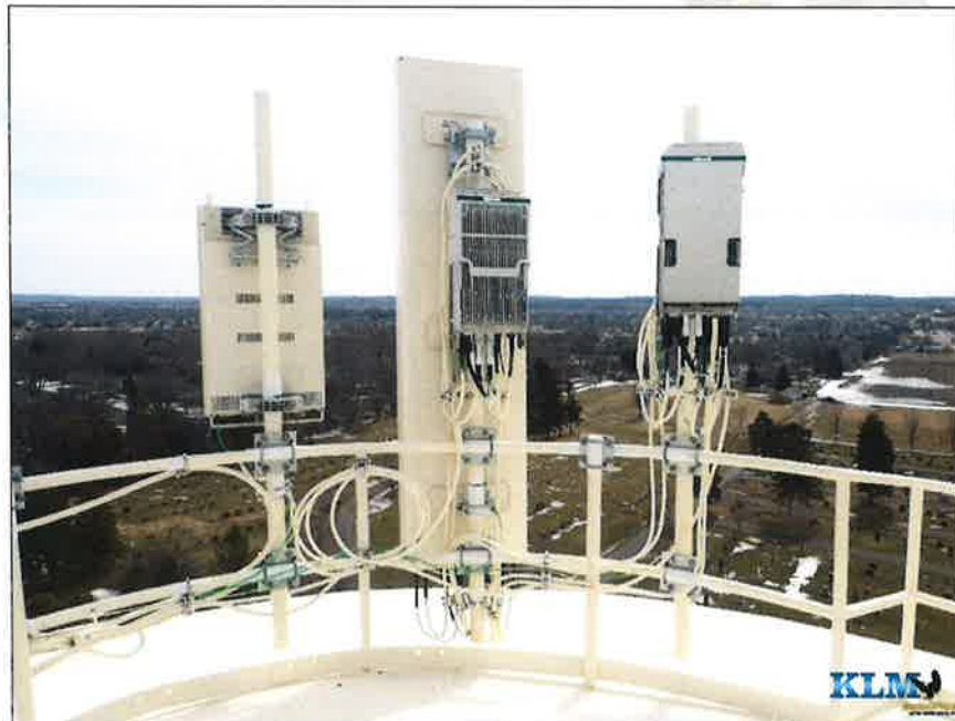
Photo No. 10 Handrail and antenna equipment
