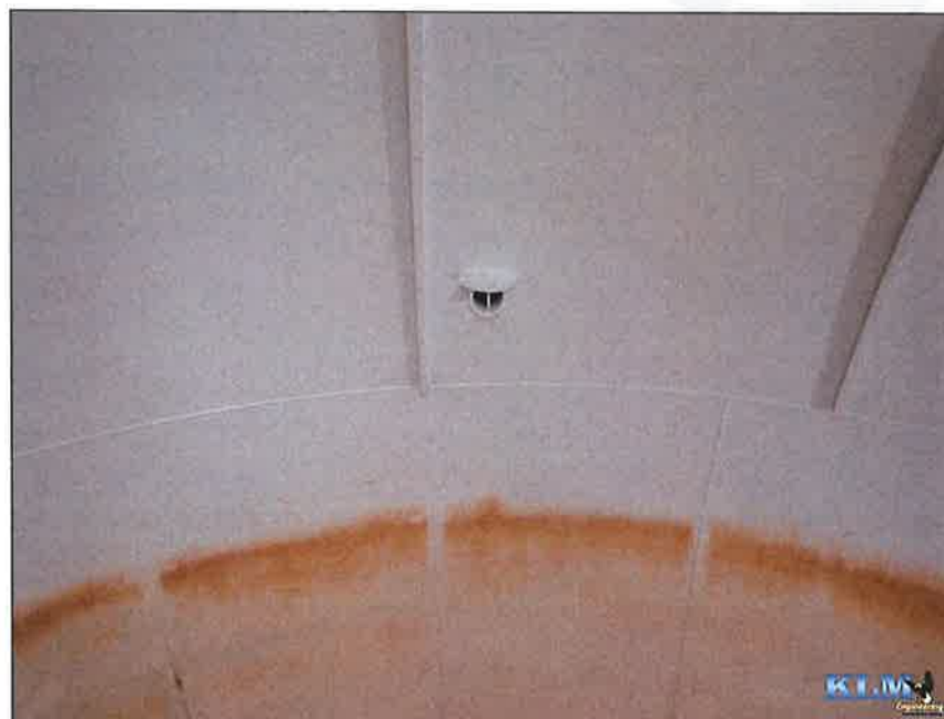
Photo No. 6 Upper torus to shell connection Overflow pipe inlet visible
