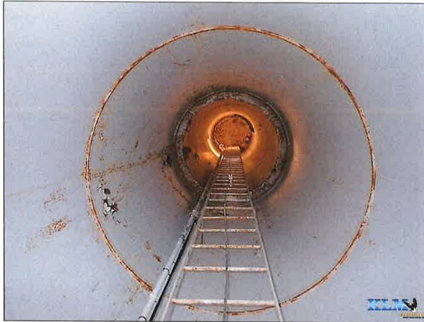
Photo No. 9 Drywell tube conditions Micro-cracking visible
