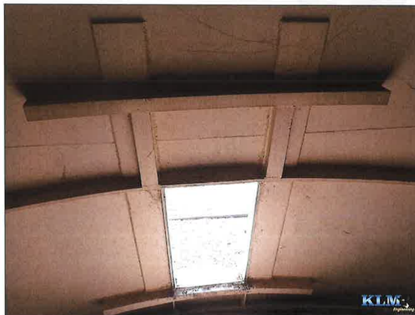
Photo No. 10 Condition of the base cone and access door reinforcement
