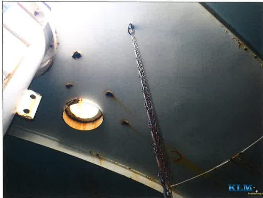
Photo No. 3 Condition of roof stiffeners and plates Mixer chain visible
