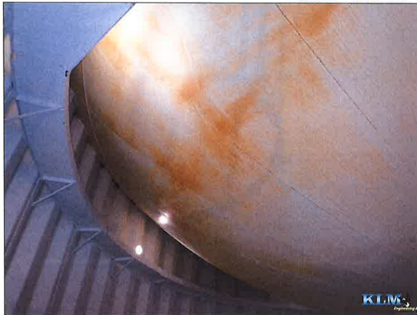
Photo No. 12 Bowl conditions with micro-cracking
