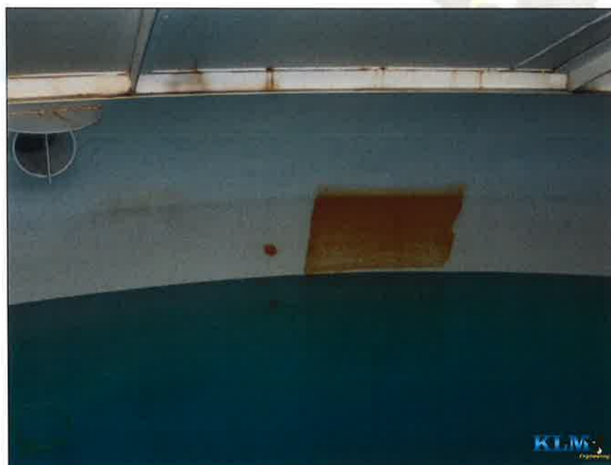
Photo No. 6 Condition of upper shell Overflow pipe inlet visible
