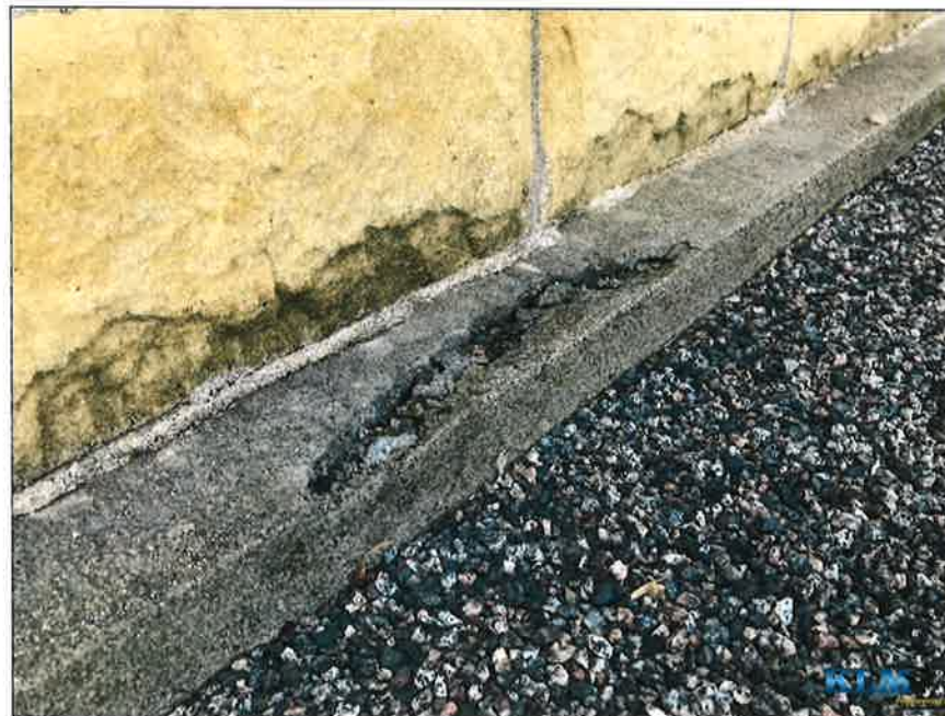
Photo No. 22 Minor spalling on foundation
