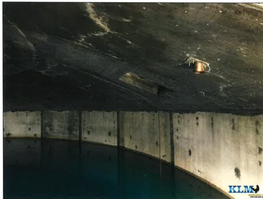
Photo No. 4 Condition of roof and wall Manway and coupling visible
