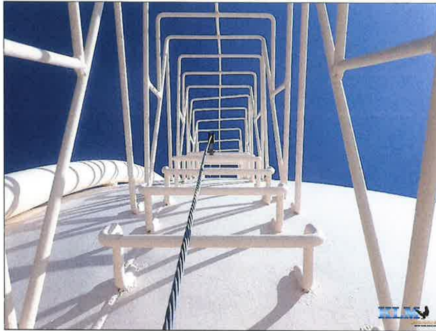
Photo No. 17 Exterior ladder and cage
