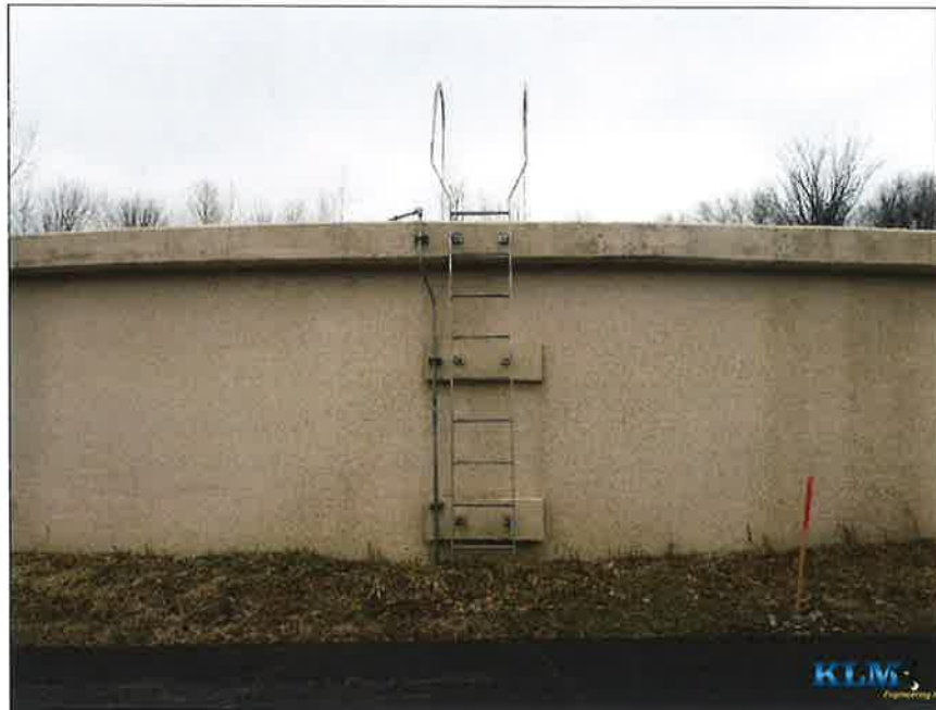
Photo No. 13 Roof access ladder
