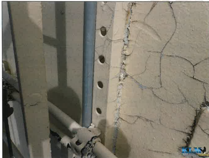
Photo No. 16 Topcoat delamination on shell
