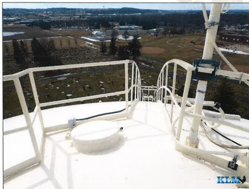
Photo No. 12 Handrail and wet access manway
