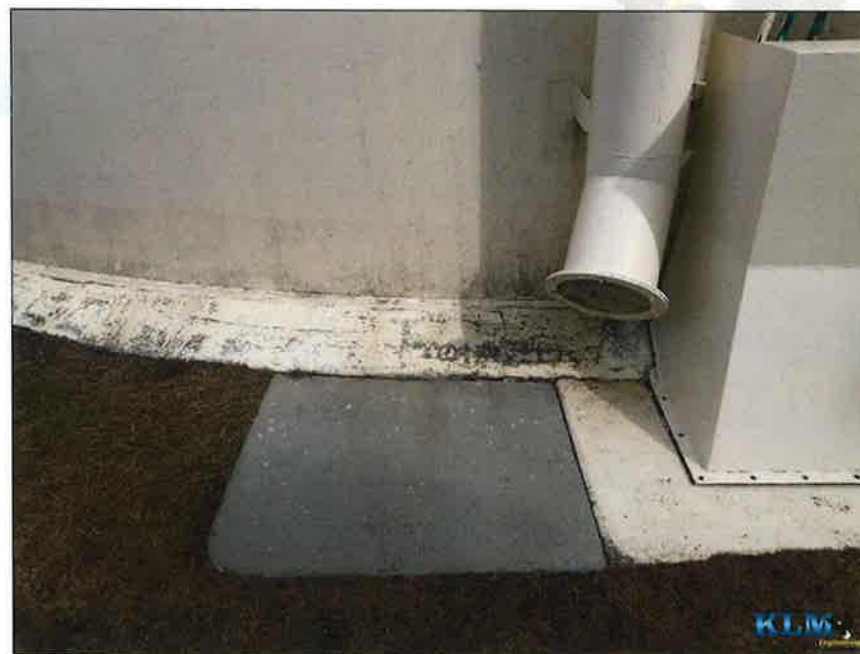
Photo No. 20 Overflow pipe and splash pad
