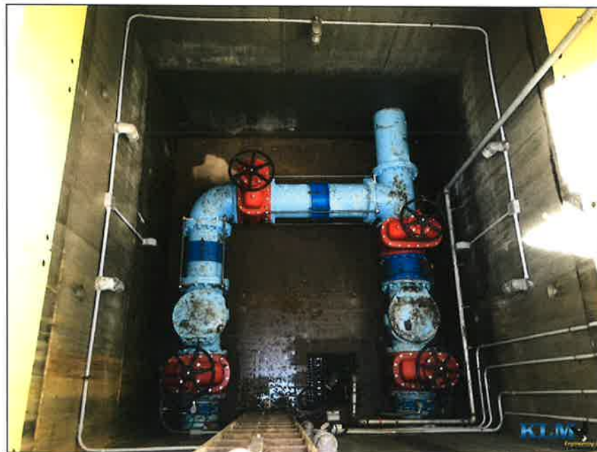
Photo No. 26 View of valve pit
