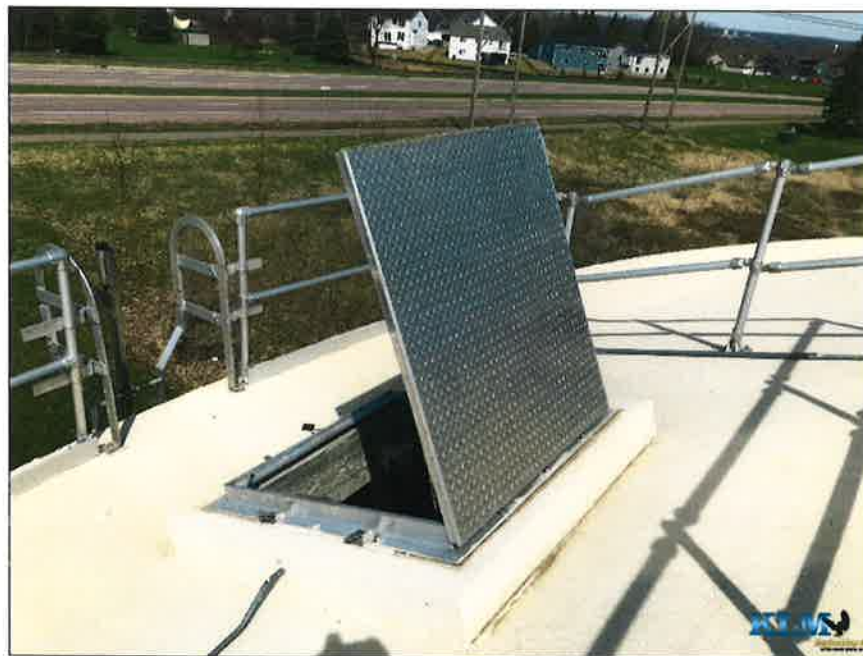
Photo No. 14 Roof hatch
