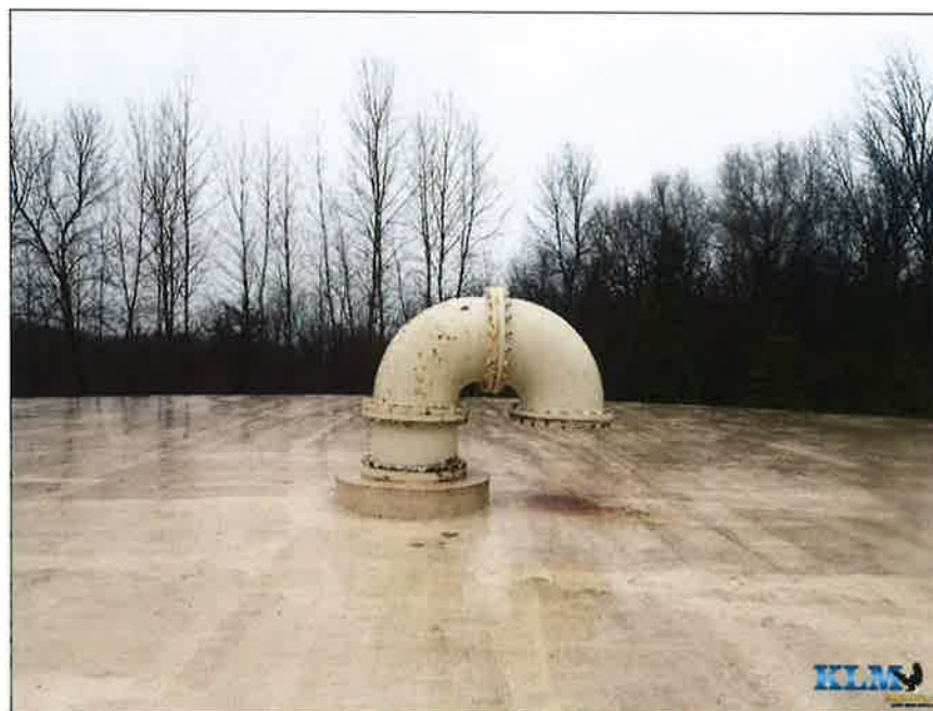
Photo No. 8 View of roof and J-vent
