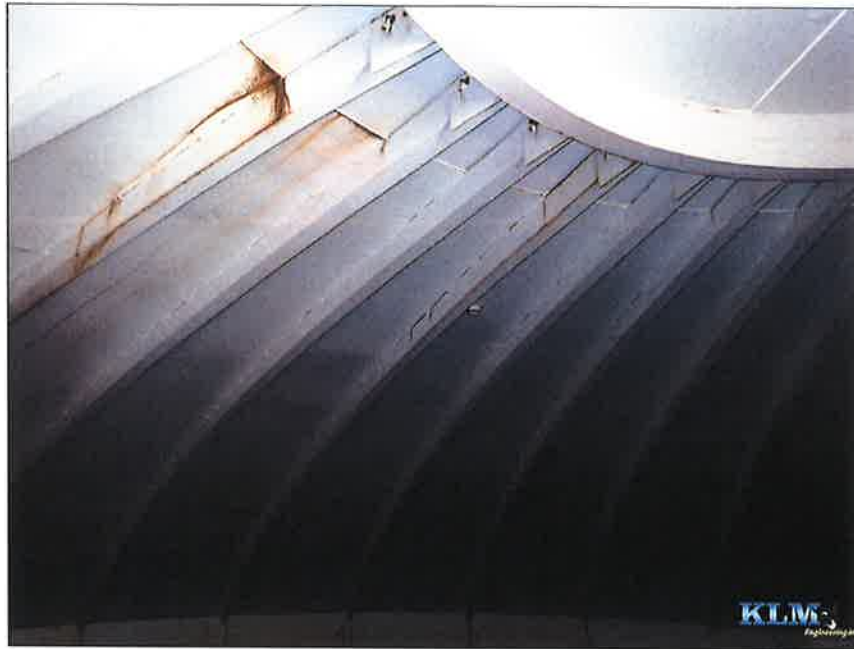
Photo No. 3 Condition of roof rafters and plates
