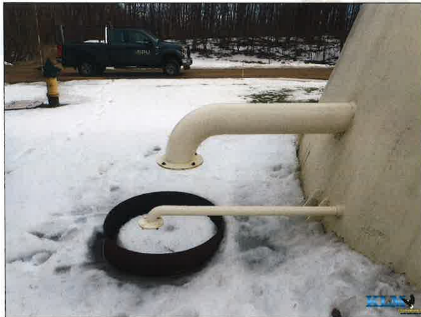
Photo No. 30 Overflow pipe and catch basin
