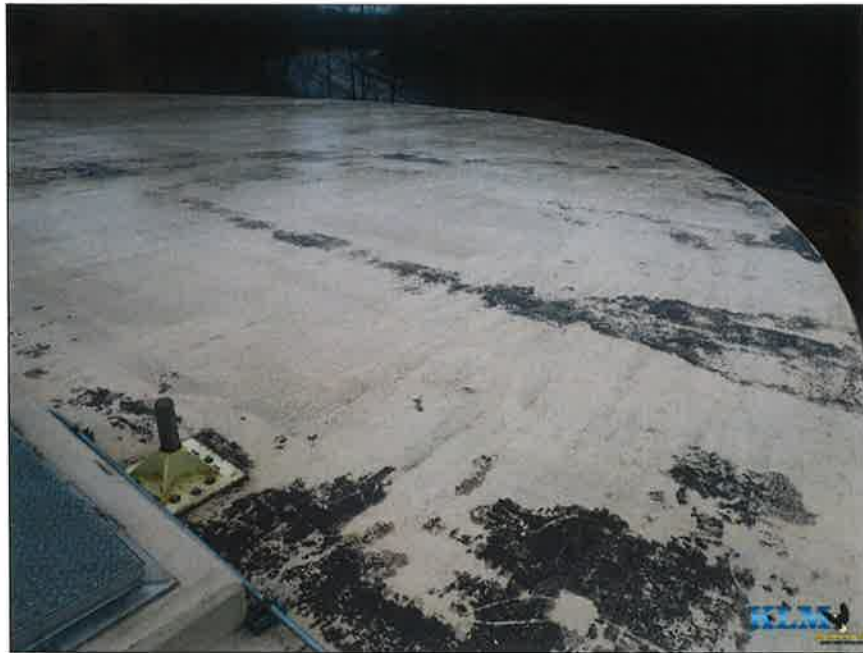
Photo No. 11 Condition of roof coating
