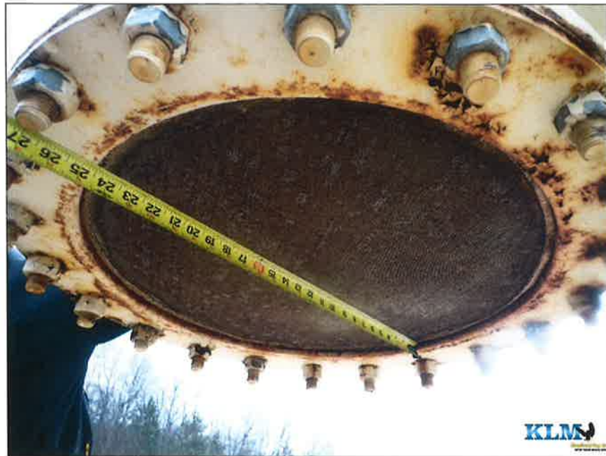
Photo No. 9 Condition of J-vent screen
