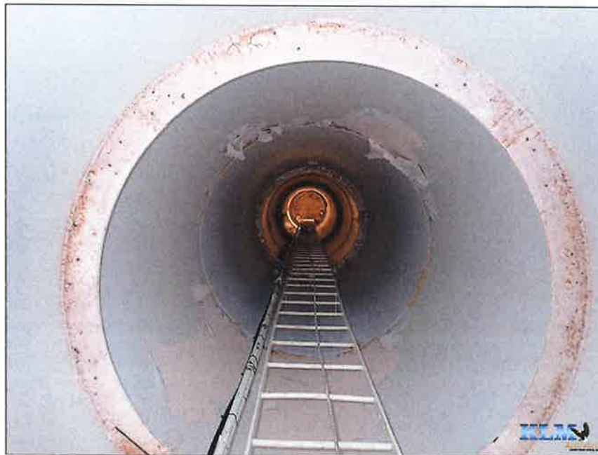
Photo No. 8 Top of drywell tube (looking down) Peeling paint visible
