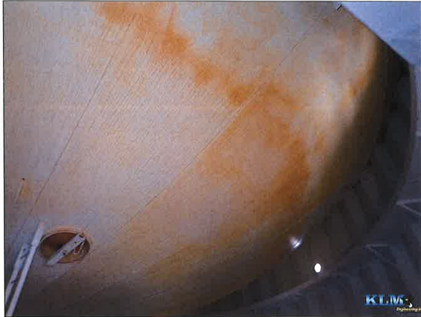
Photo No. 13 Bowl conditions with micro-cracking
