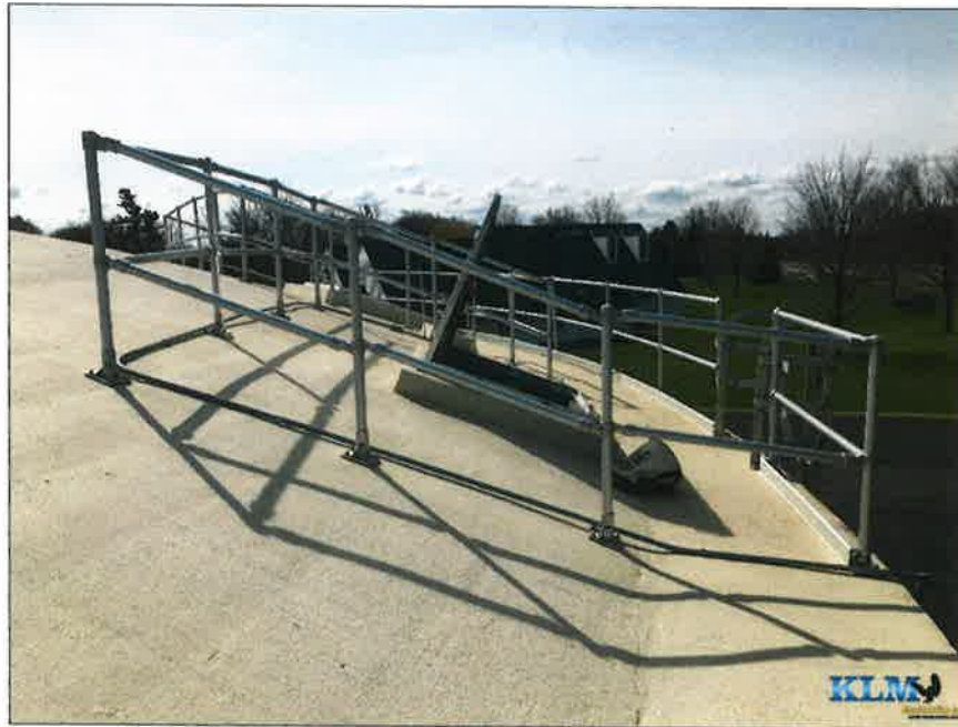
Photo No. 13 Roof handrailing
