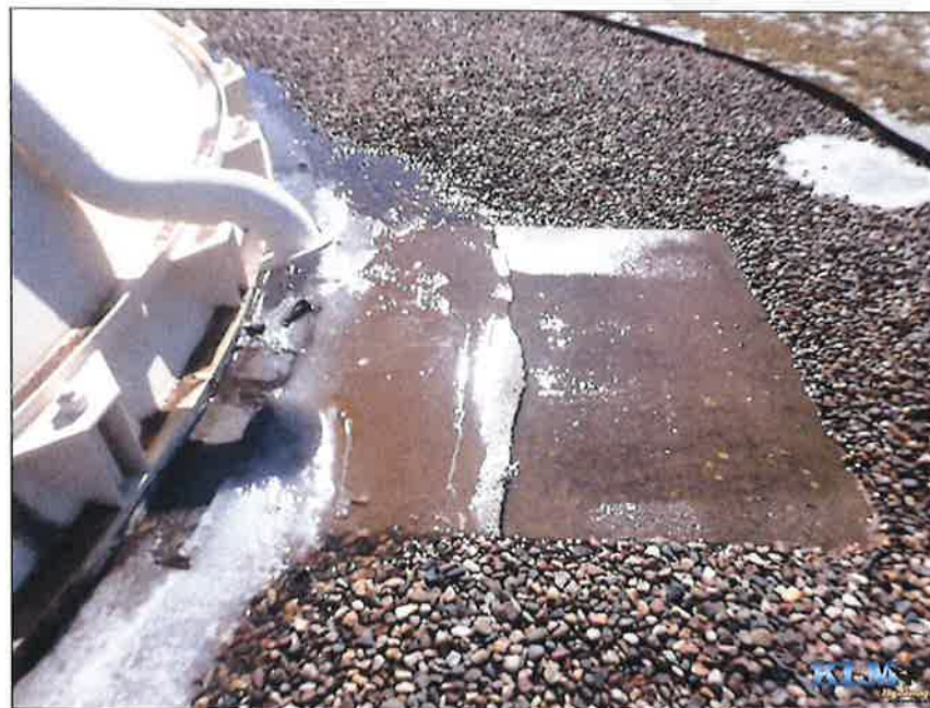
Photo No. 22 Overflow pipe outlet and splash pad
