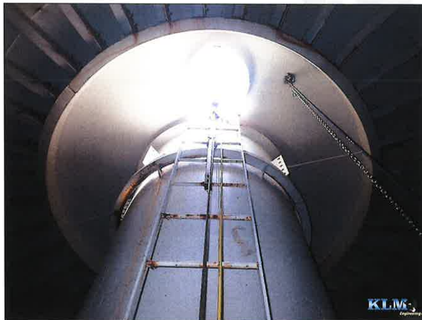
Photo No. 2 Interior wet ladder and dollar plate
