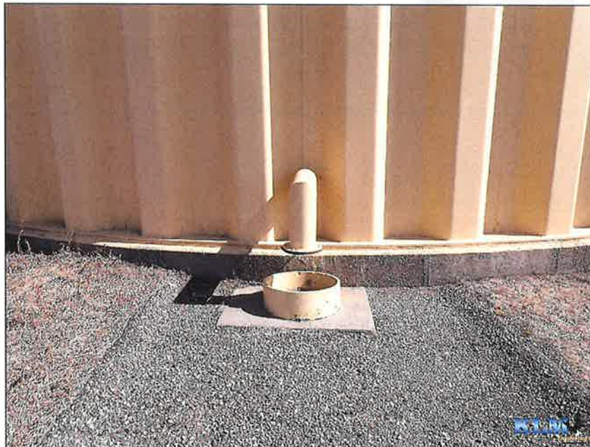
Photo No. 28 Overflow pipe and catch basin
