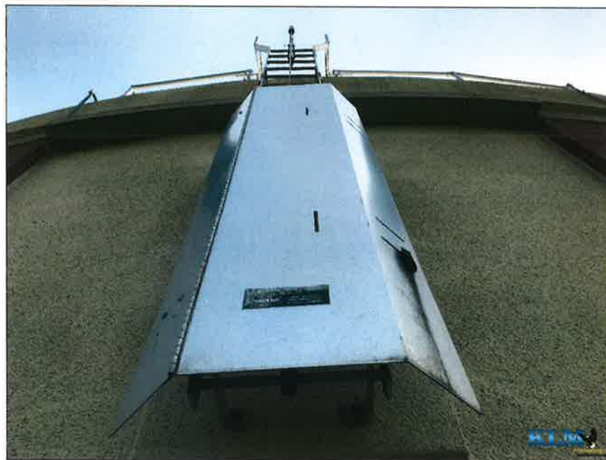
Photo No. 16 Access ladder with anti-climb plate
