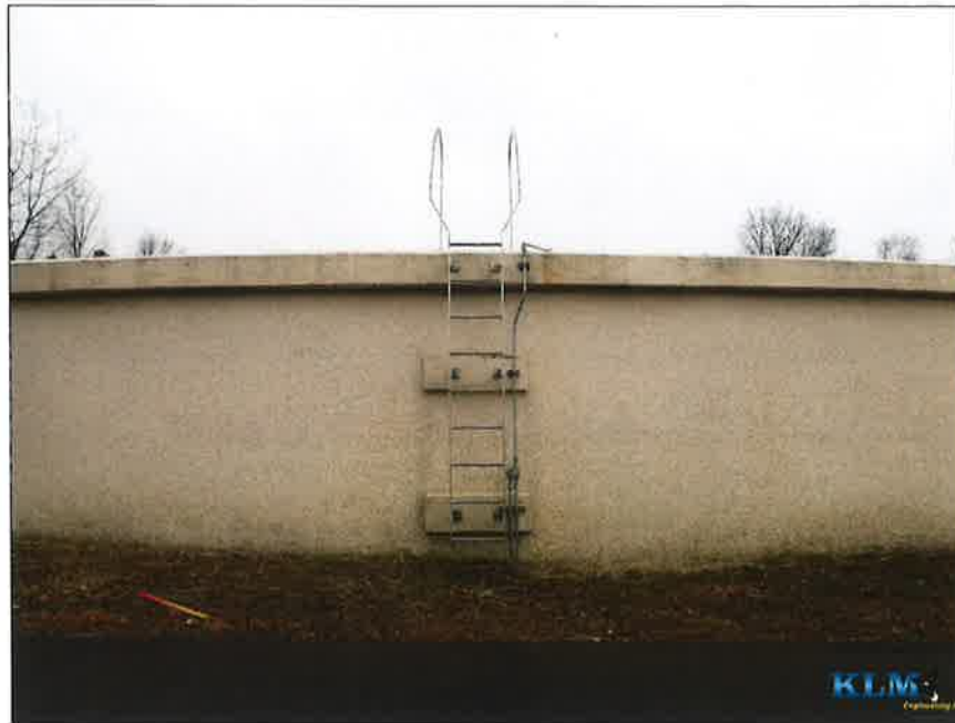
Photo No. 13 Roof access ladder
