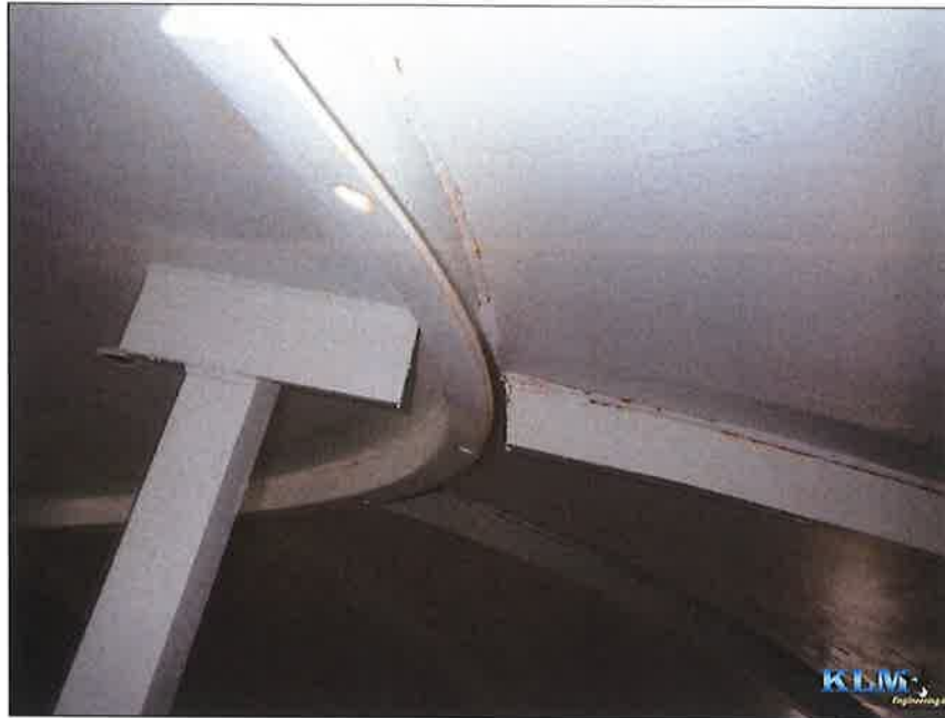
Photo No. 3 Condition of compression ring and rafters
