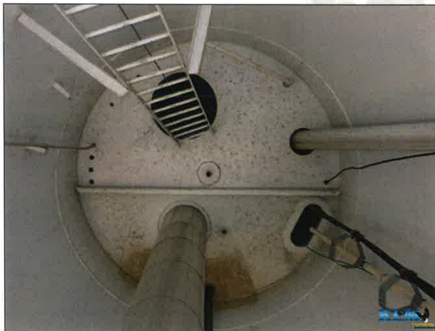
Photo No. 16 Underside of bottom landing
