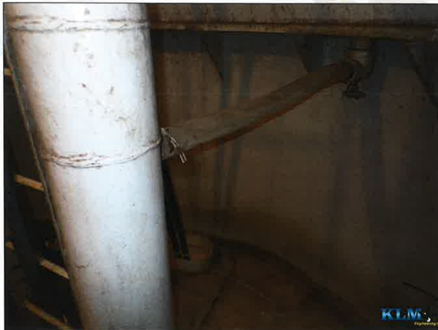
Photo No. 12 Bowl drain valve and connecting line
