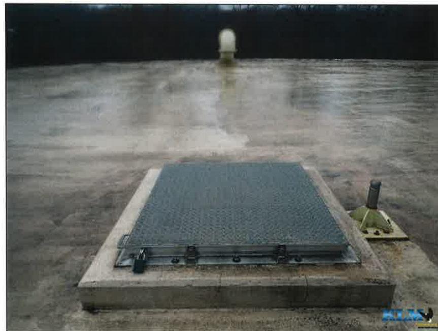
Photo No. 12 Bilco access hatch
