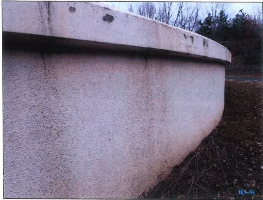
Photo No. 13 Typical wall condition
