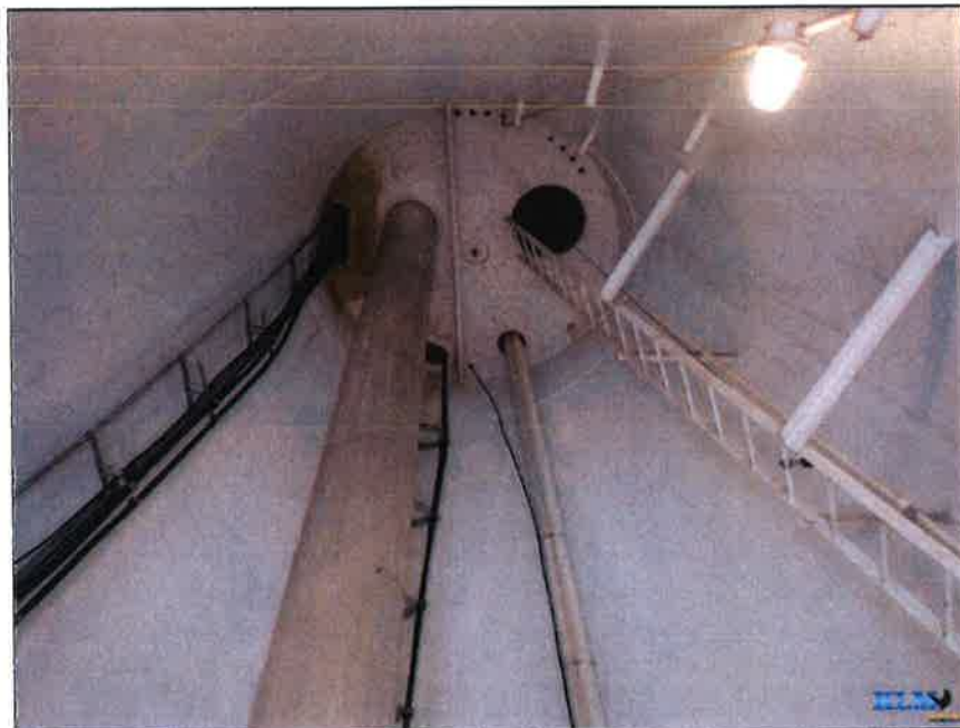
Photo No. 16 Base cone conditions
