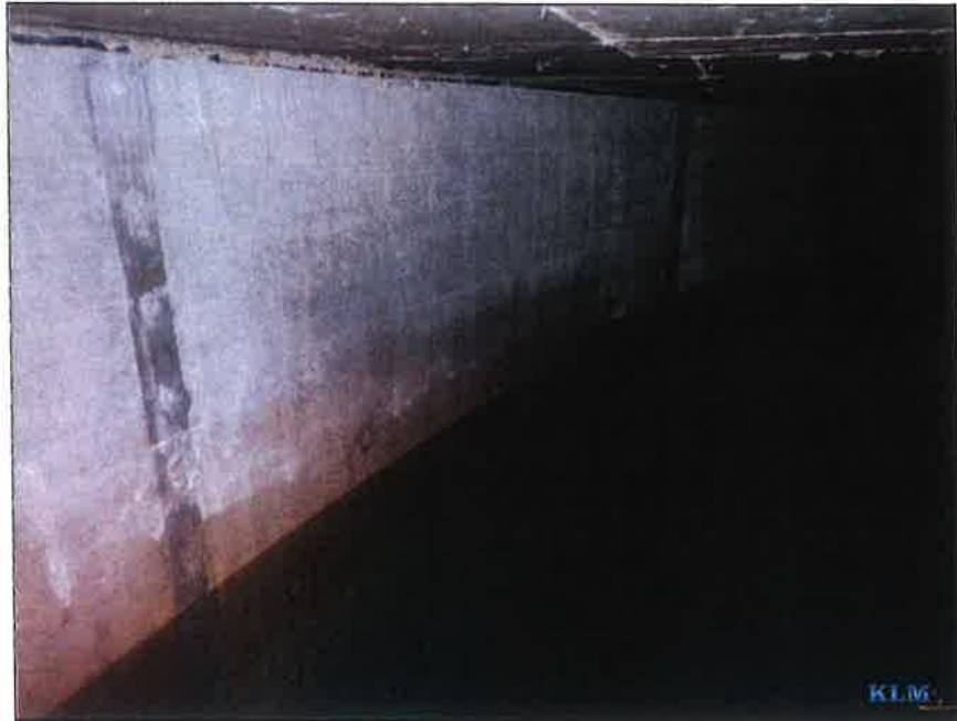
Photo No. 5 Condition of roof and wall
