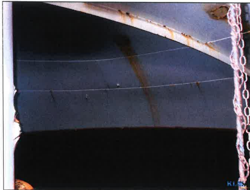
Photo No. 6 Condition of roof and upper torus
