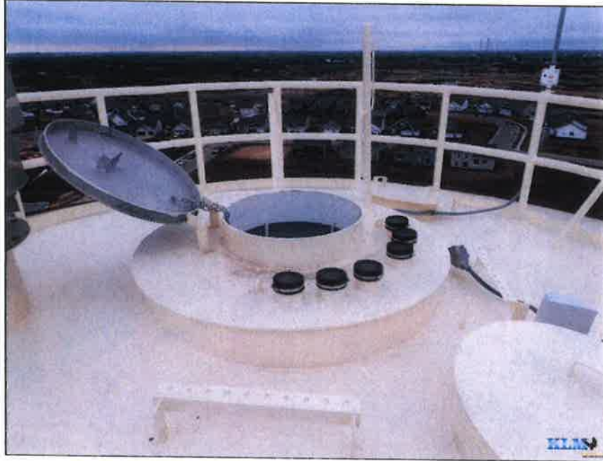
Photo No. 37 Drywell tube manway
