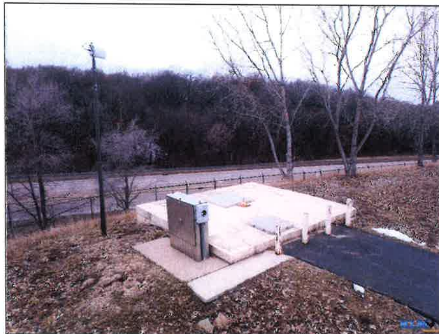
Photo No. 18 Exterior view of valve pit
