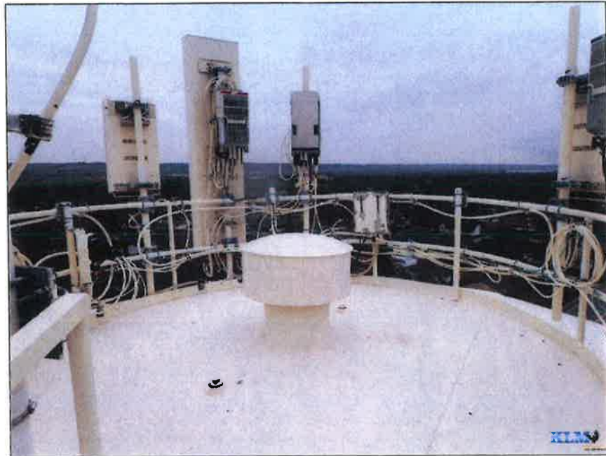
Photo No. 7 Overall conditions on roof
