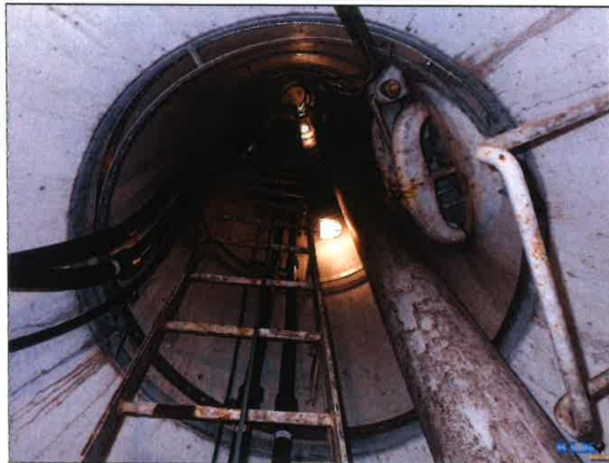
Photo No. 10 Overall conditions in drywell tube
