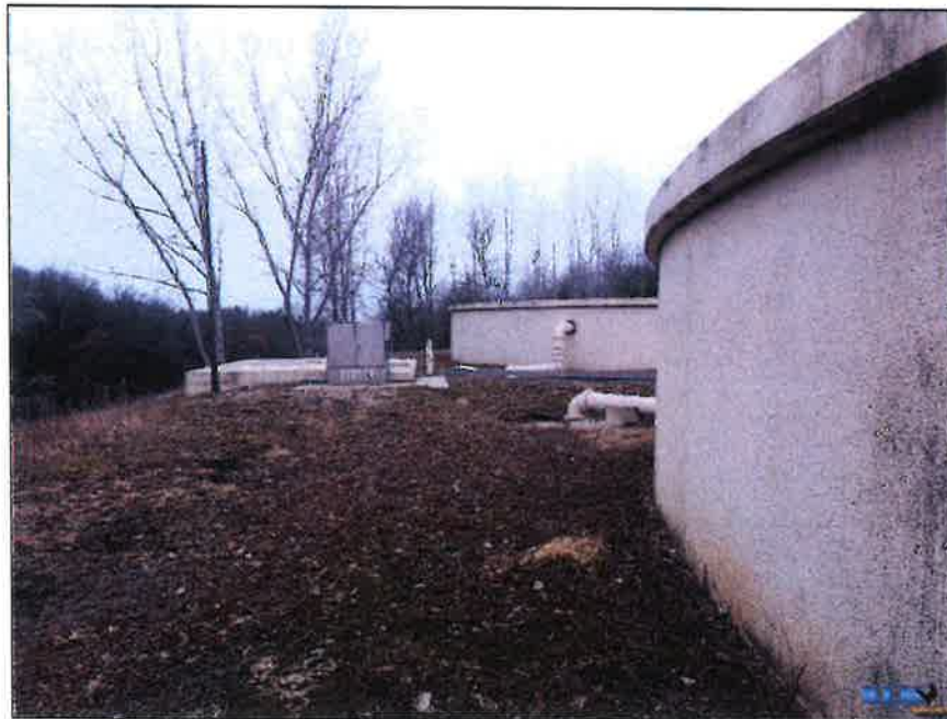
Photo No. 14 Typical wall condition
