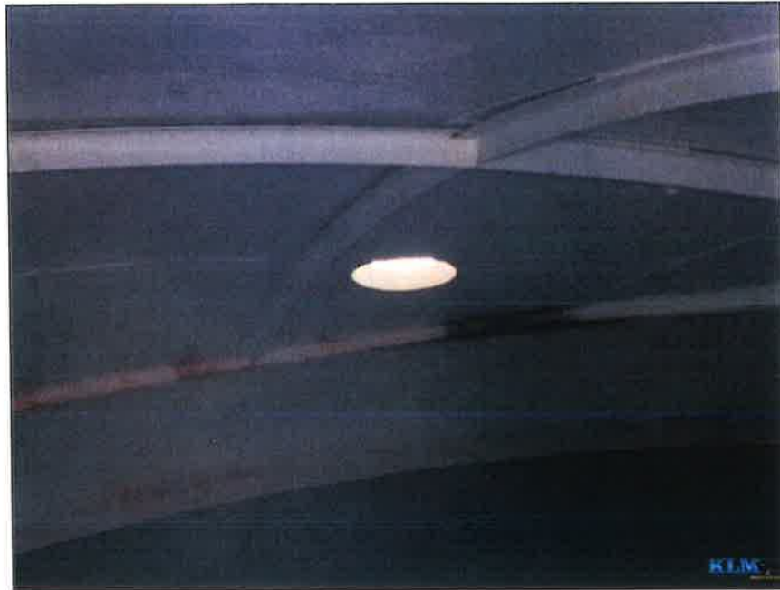
Photo No. 3 Interior roof conditions
