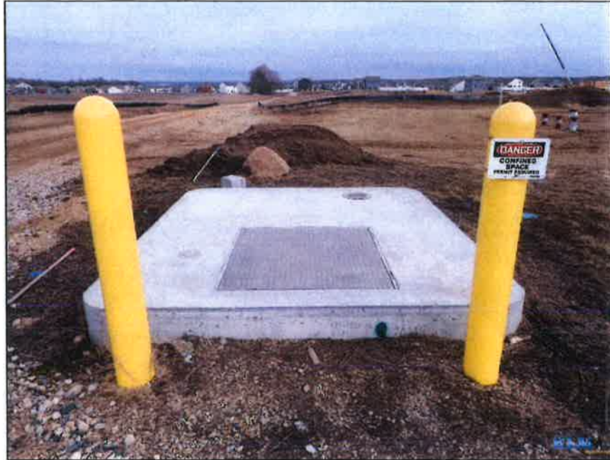
Photo No. 51 Valve pit manway
