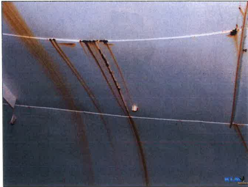
Photo No. 3 Overall condition of roof
