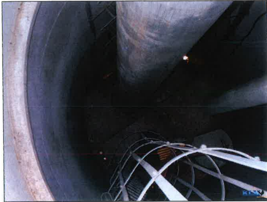
Photo No. 15 Overall conditions in riser
