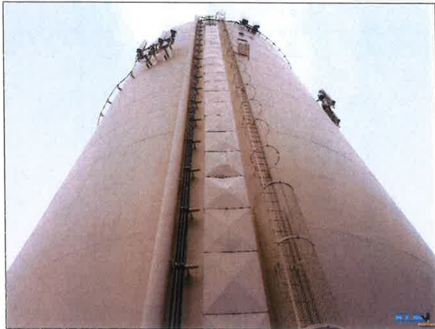
Photo No. 17 Ladder and condition of shell
