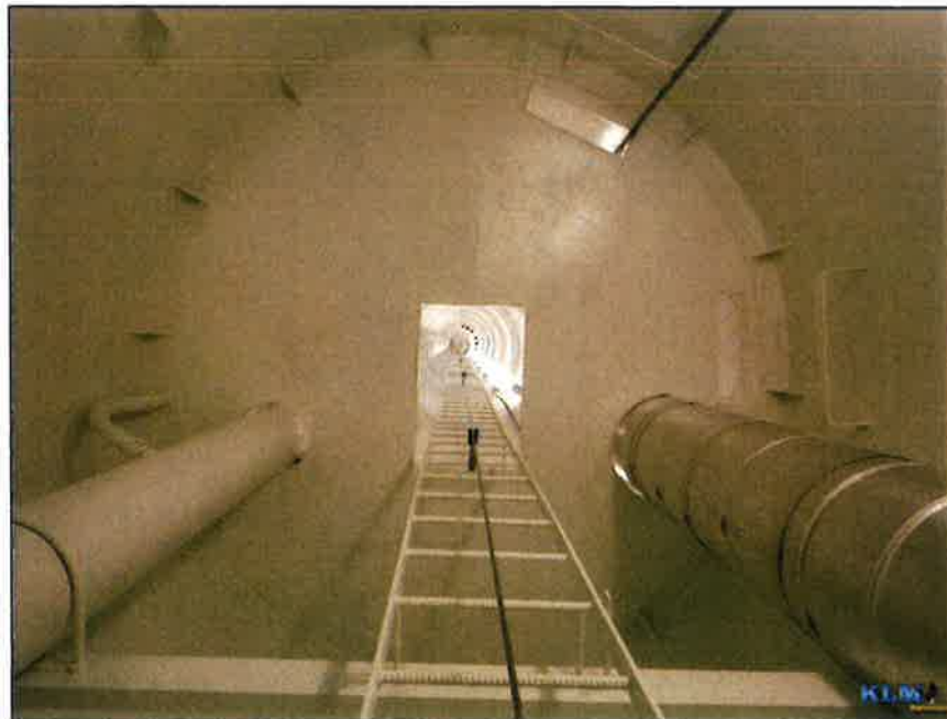
Photo No. 32 Underside of top landing
