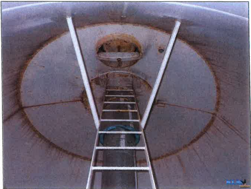
Photo No. 9 Base cone to wet riser transition
