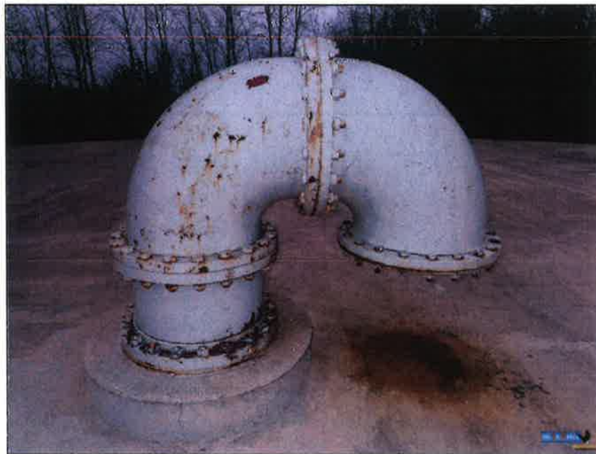
Photo No. 8 Condition of J-vent
