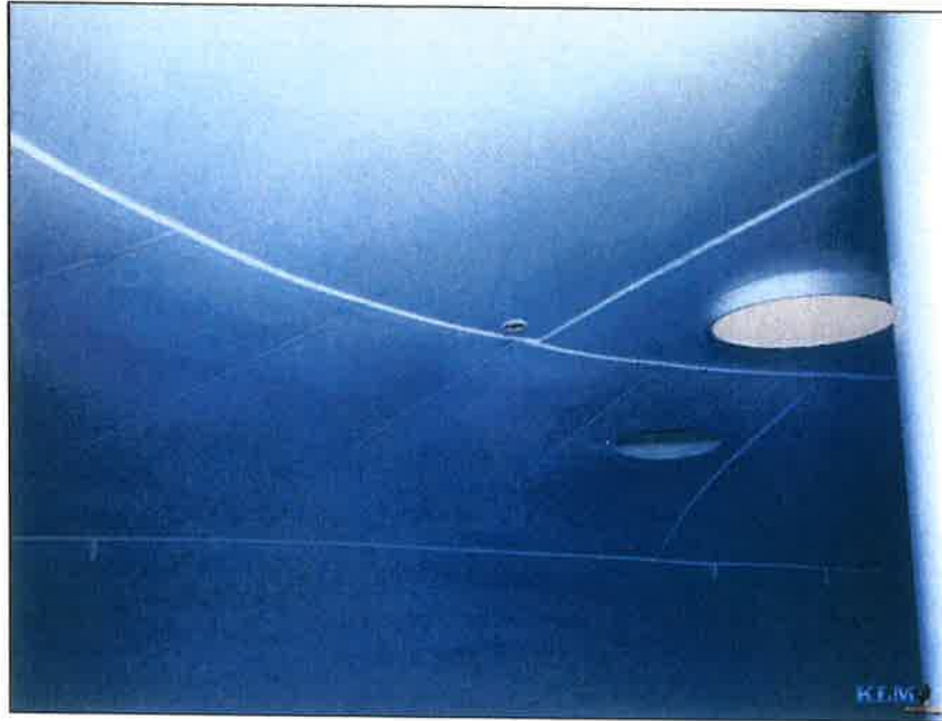
Photo No. 5 Roof coating conditions
