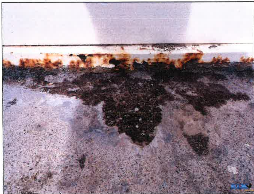
Photo No. 24 Base plate and foundation conditions
