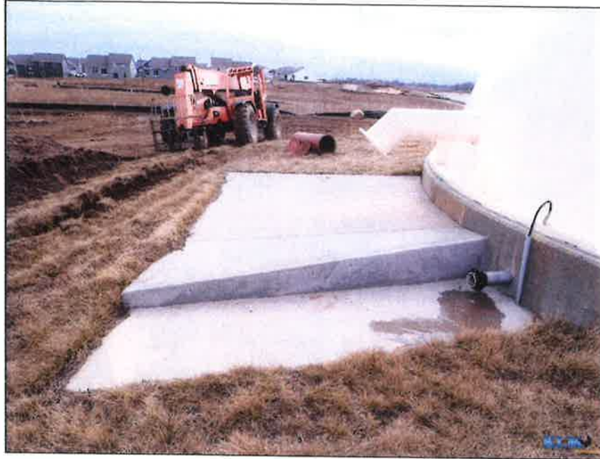
Photo No. 49 Overflow pipe outlet and splash pad
