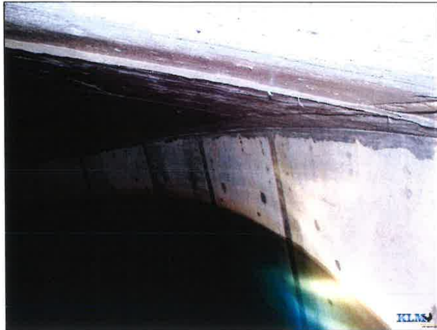
Photo No. 3 Typical condition of roof and wall
