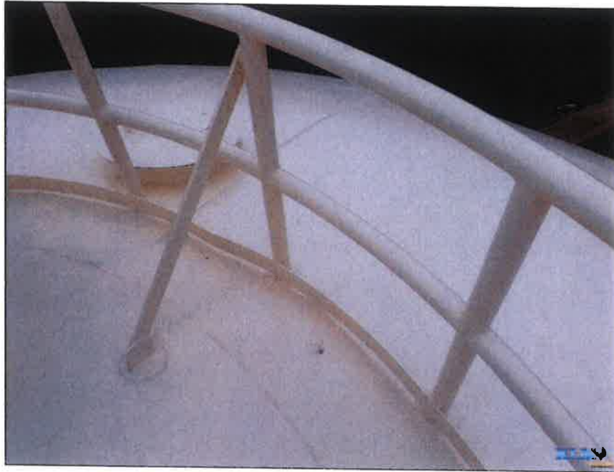
Photo No. 41 Handrail coating conditions
