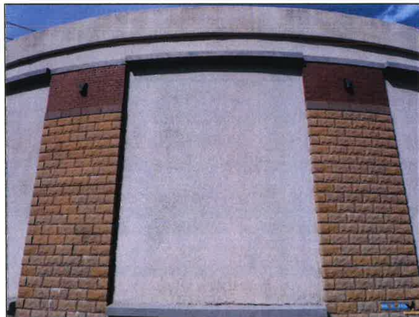
Photo No. 16 Condition of wall
