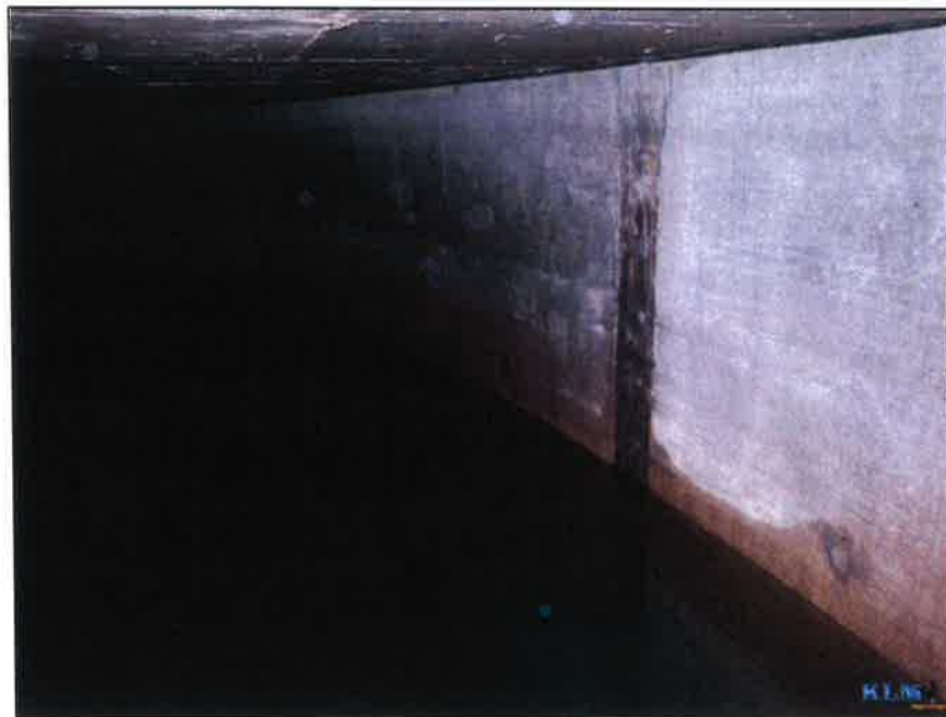
Photo No. 6 Condition of wall
