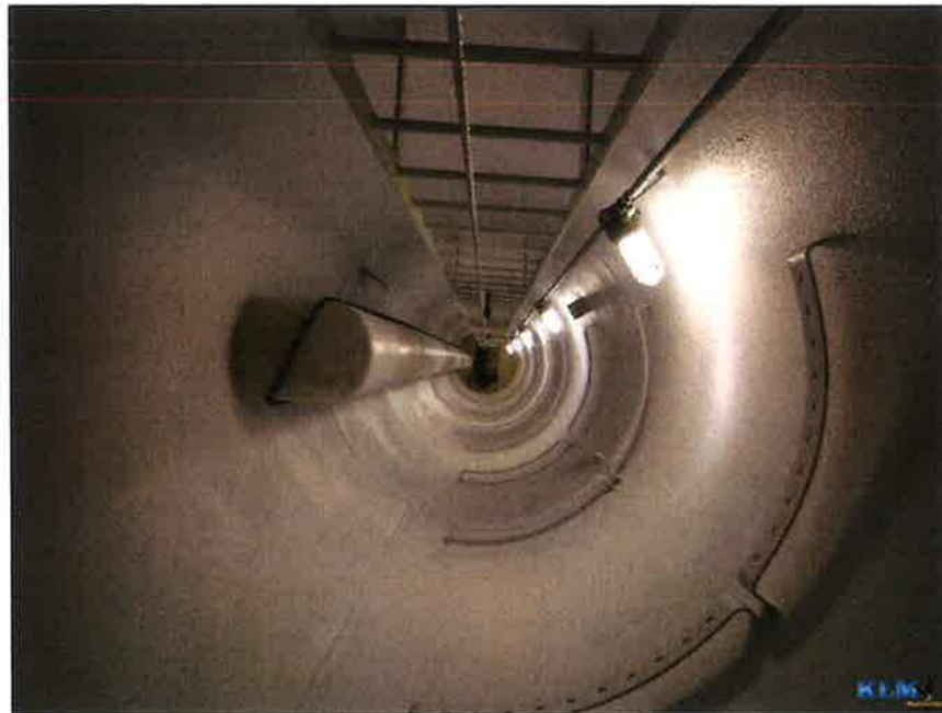
Photo No. 24 Top of drywell tube (looking down)
