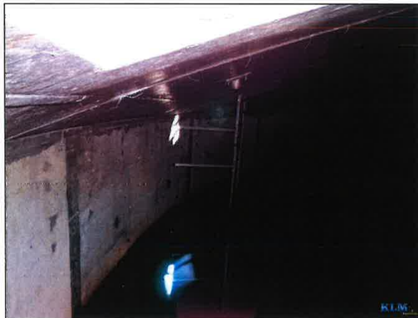
Photo No. 4 Roof, wall, and ladder conditions
