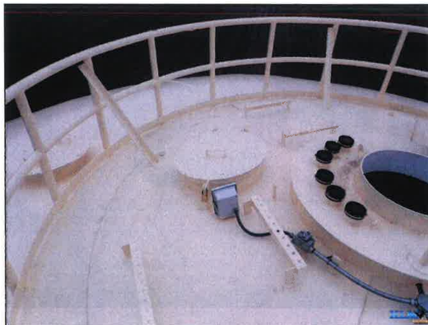
Photo No. 40 Roof conditions
