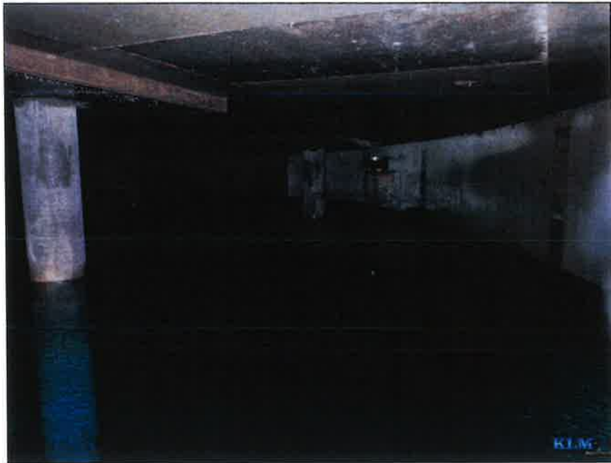
Photo No. 7 Condition of column with overflow in background
