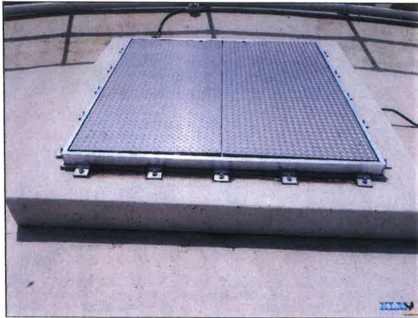
Photo No. 13 Roof hatch
