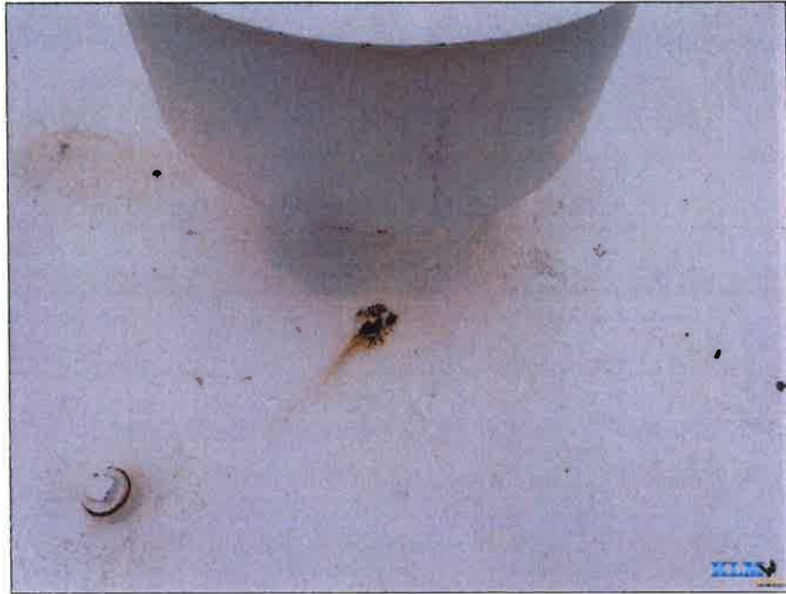
Photo No. 11 Coating conditions on roof
