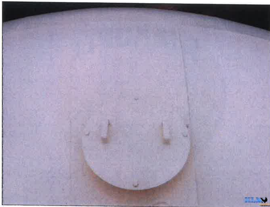
Photo No. 42 Roof plate coating conditions Ventilation manway visible
