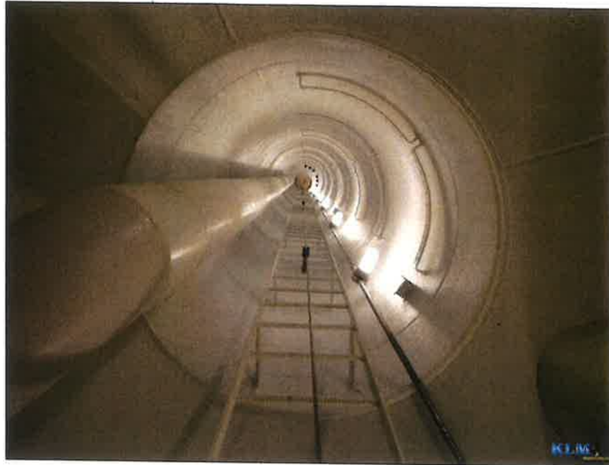
Photo No. 25 Bottom of drywell tube (looking up)
