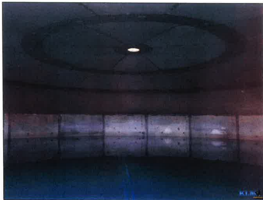
Photo No. 6 View of roof and wall
