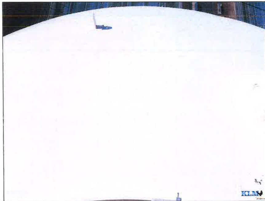
Photo No. 16 Roof coating conditions
