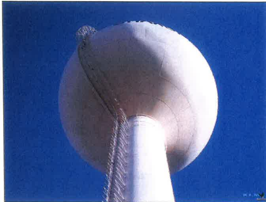
Photo No. 17 Overall condition of water compartment
