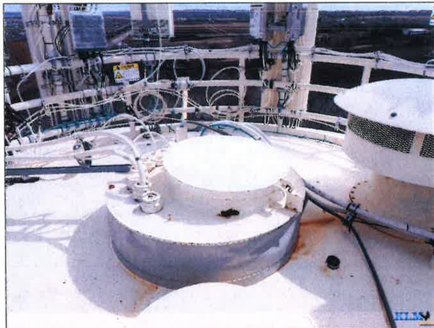
Photo No. 20 Conditions on roof
