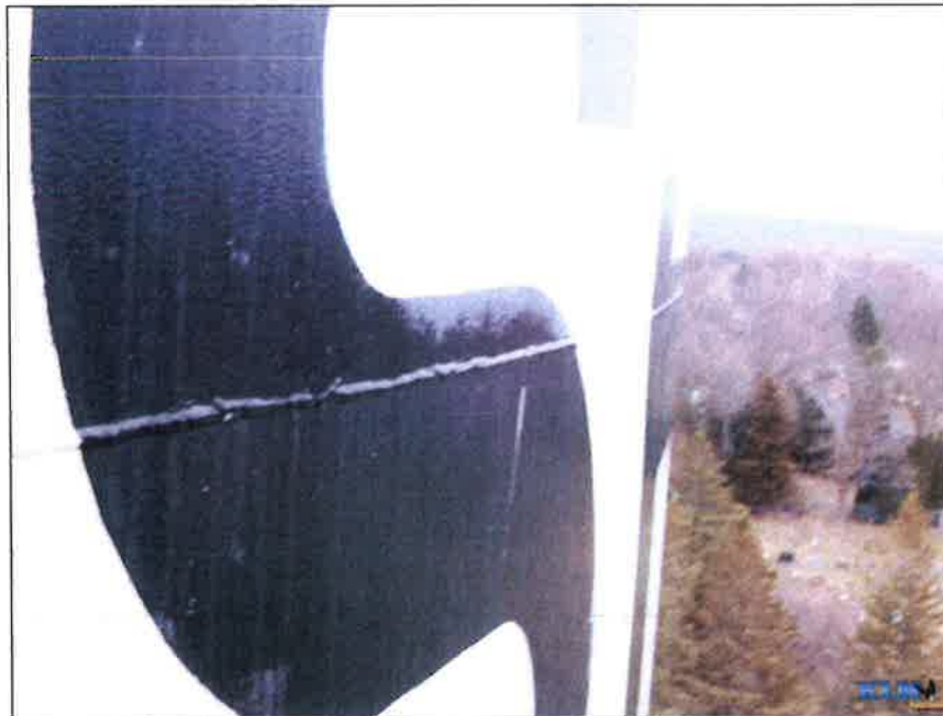
Photo No. 16 Coating condition of shell
