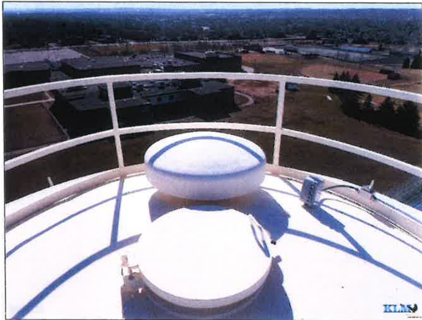
Photo No. 13 Conditions on roof
