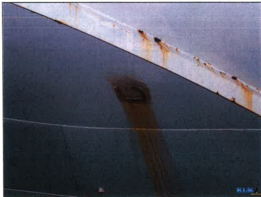
Photo No. 4 Overall condition of roof
