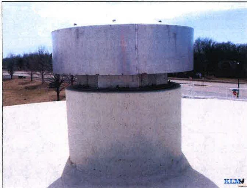
Photo No. 8 Finial vent
