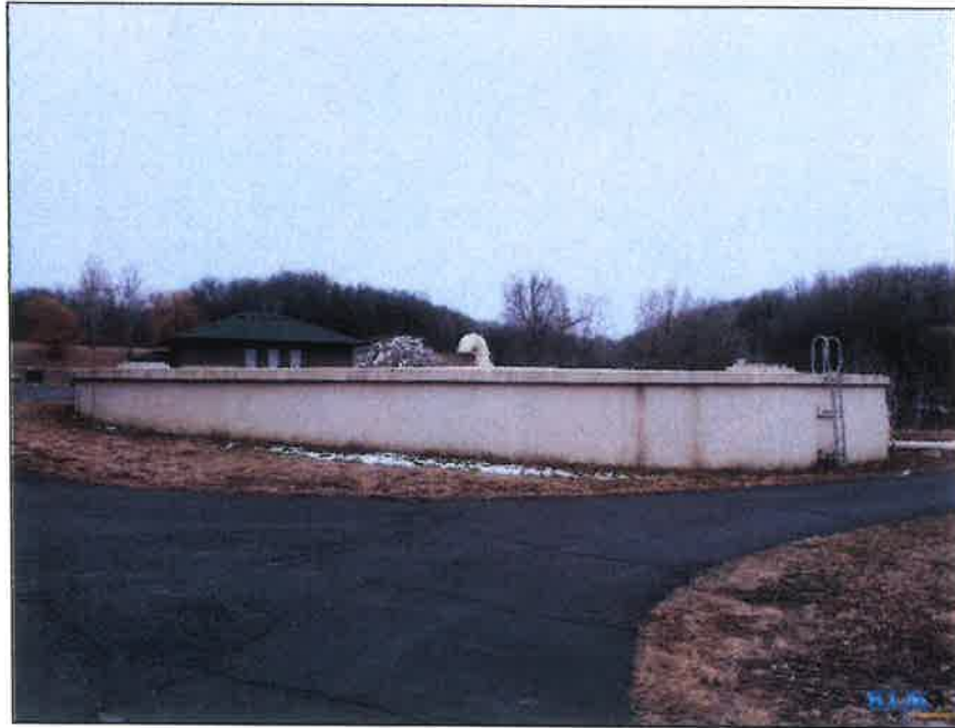
Photo No. 1 Overall view of reservoir
