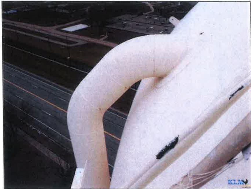
Photo No. 13 Upper torus and overflow pipe penetration
