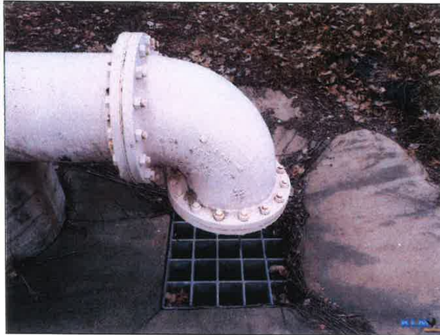
Photo No. 17 Condition of overflow pipe and grating
