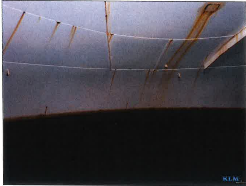
Photo No. 5 Condition of roof and upper torus
