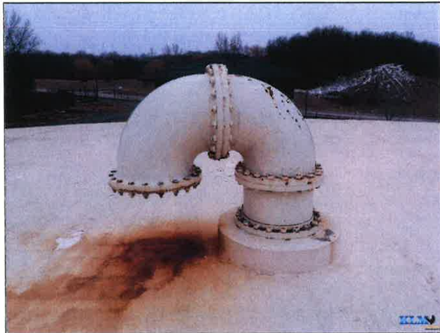
Photo No. 8 Condition of J-vent
