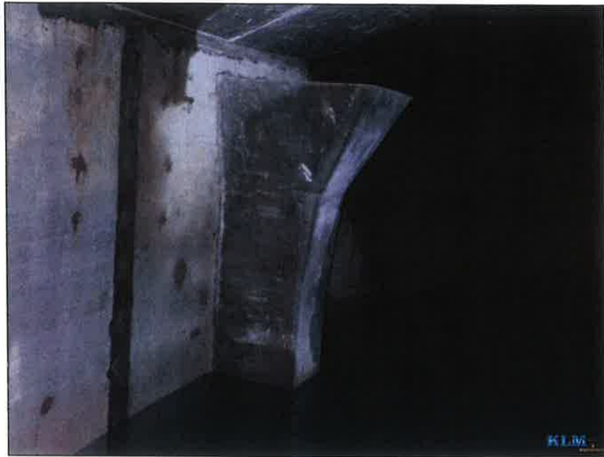
Photo No. 5 Condition of wall Overflow weir box visible
