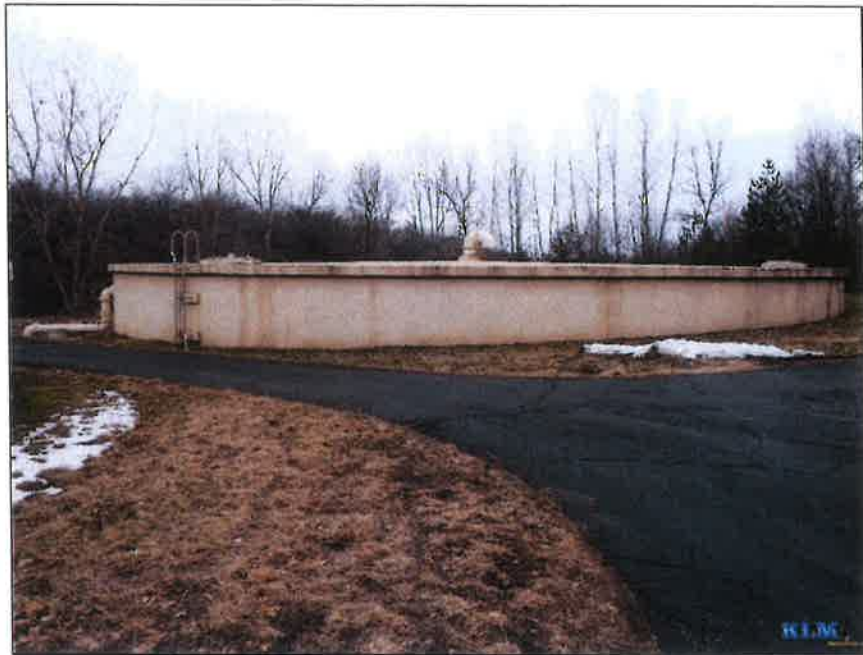
Photo No. 1 Overall view of reservoir
