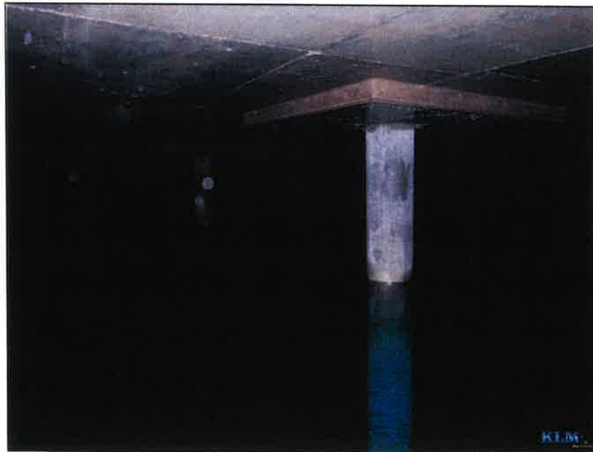
Photo No. 2 View of interior roof and column
