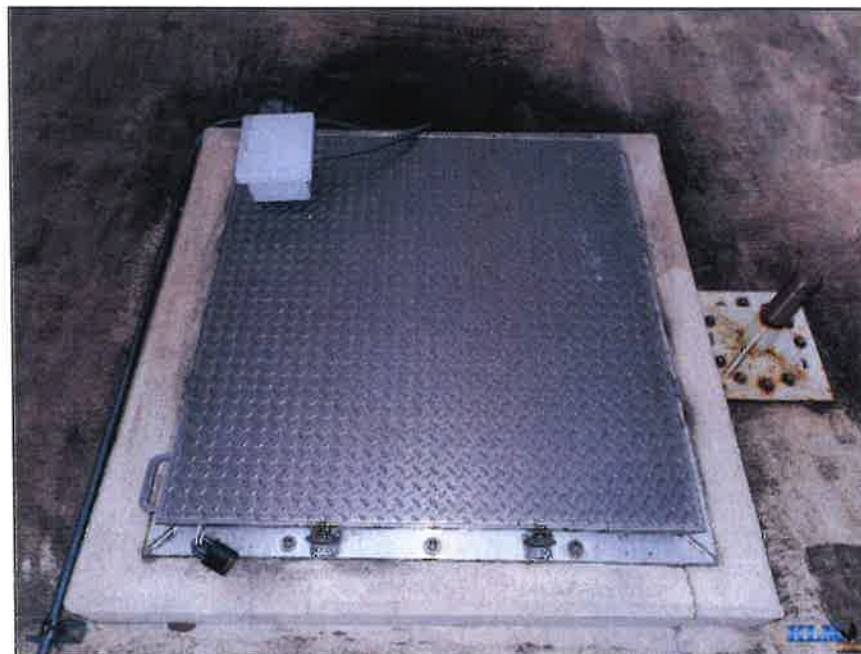
Photo No. 10 Condition of roof hatch
