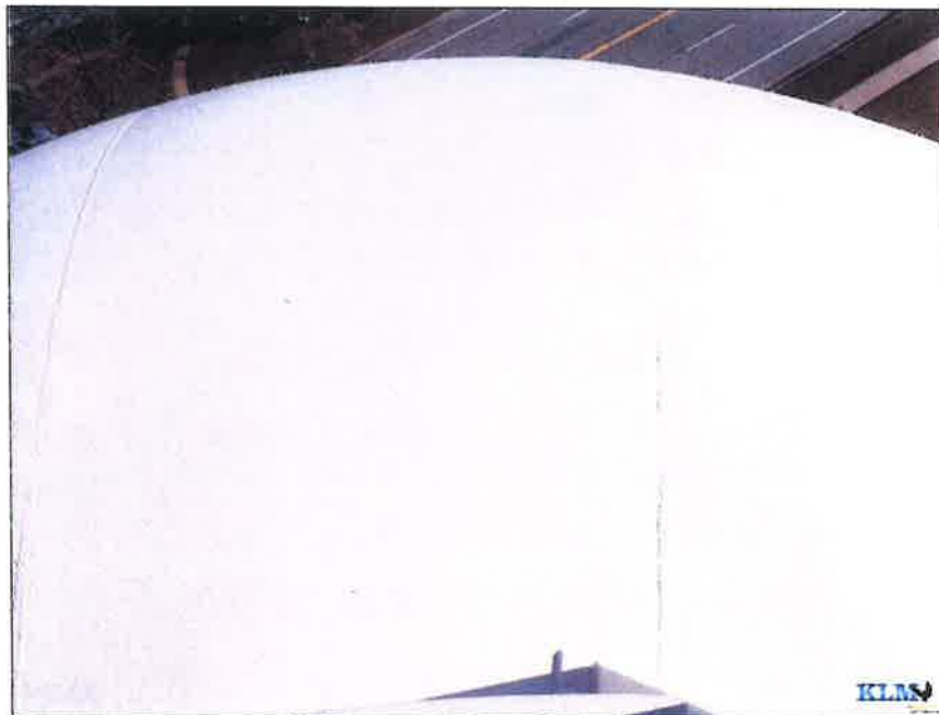
Photo No. 14 Roof coating conditions
