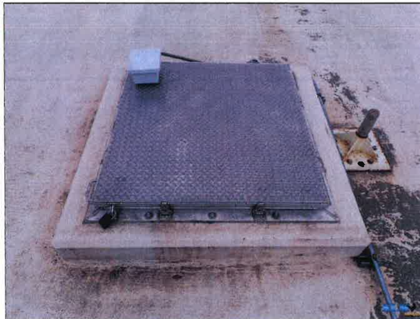
Photo No. 12 Bilco access hatch
