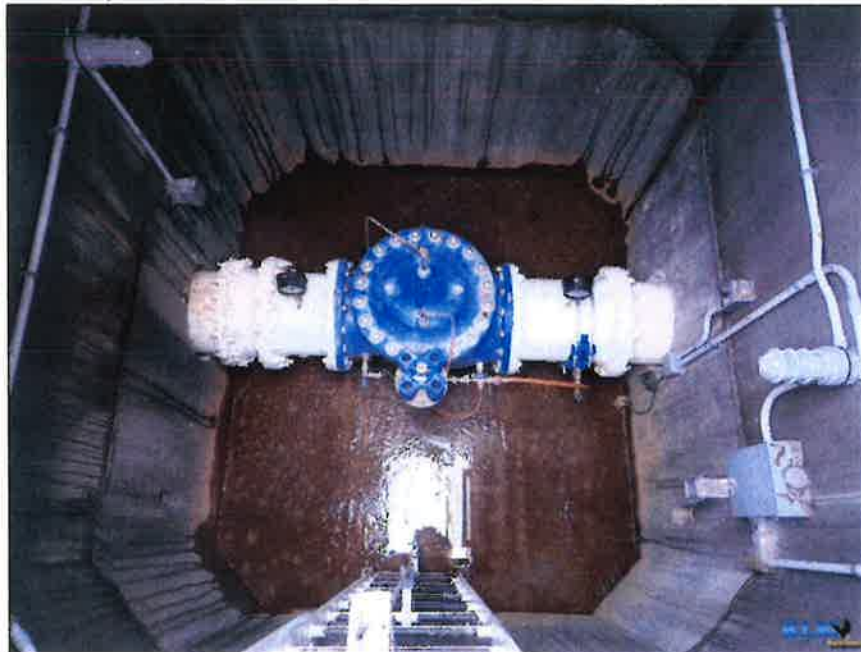
Photo No. 52 Valve pit conditions
