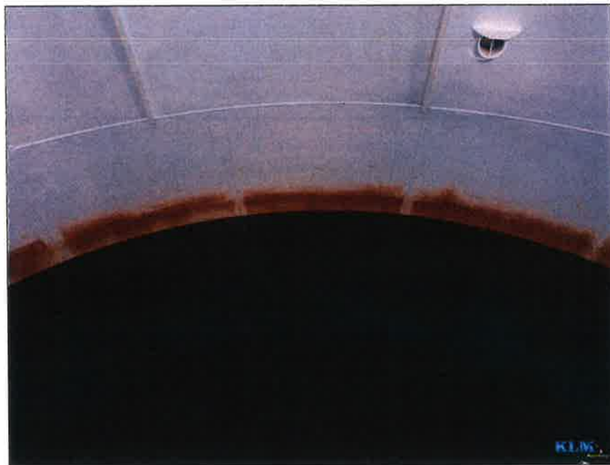
Photo No. 4 Upper torus and shell condition
