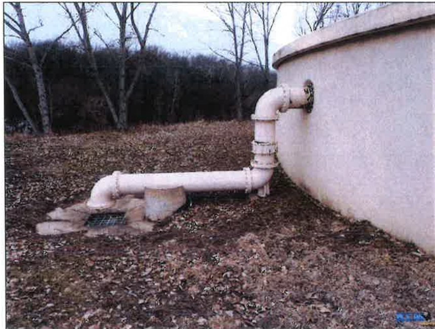
Photo No. 15 Overflow pipe and catch basin
