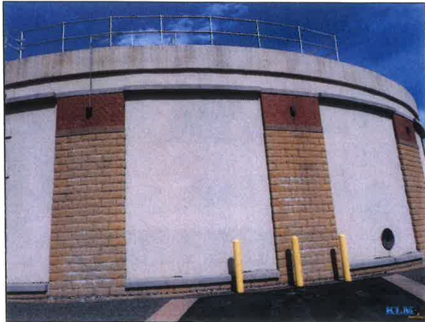
Photo No. 17 Condition of wall
