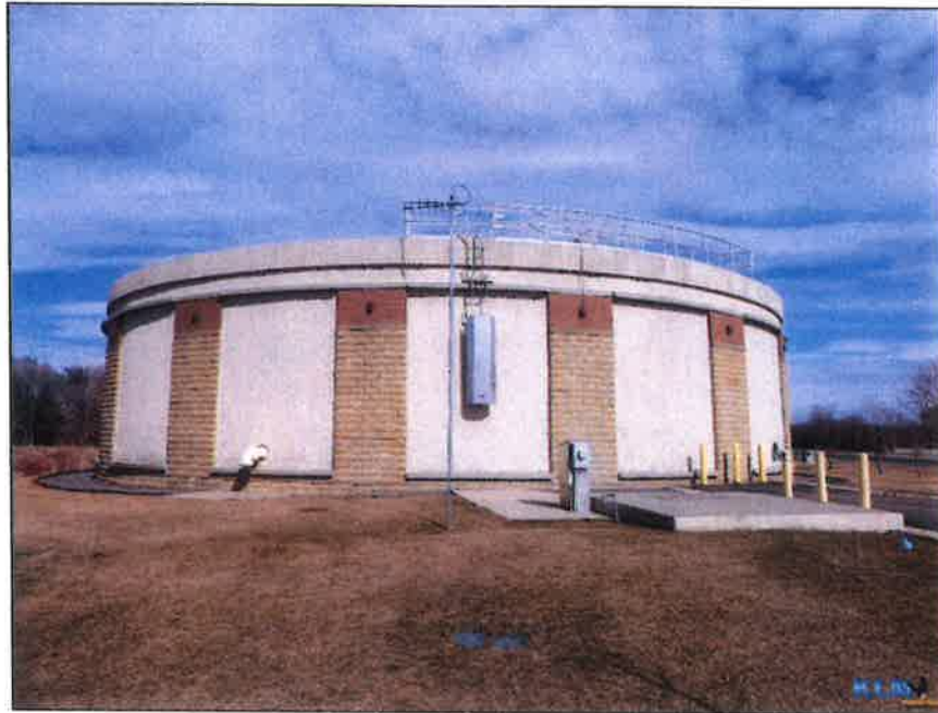
Photo No. 1 Overall view of reservoir
