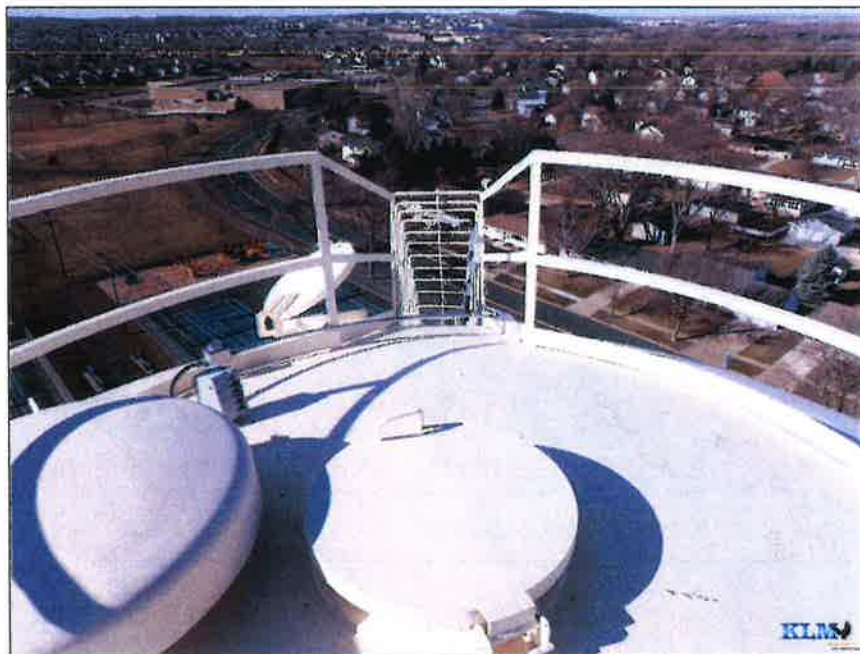
Photo No. 12 Conditions on roof
