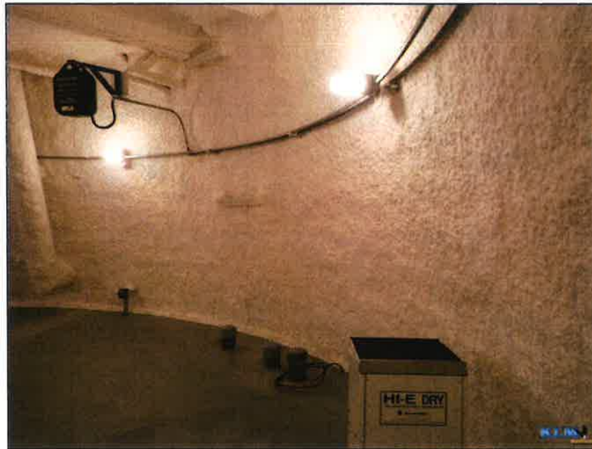
Photo No. 36 Base cone conditions
