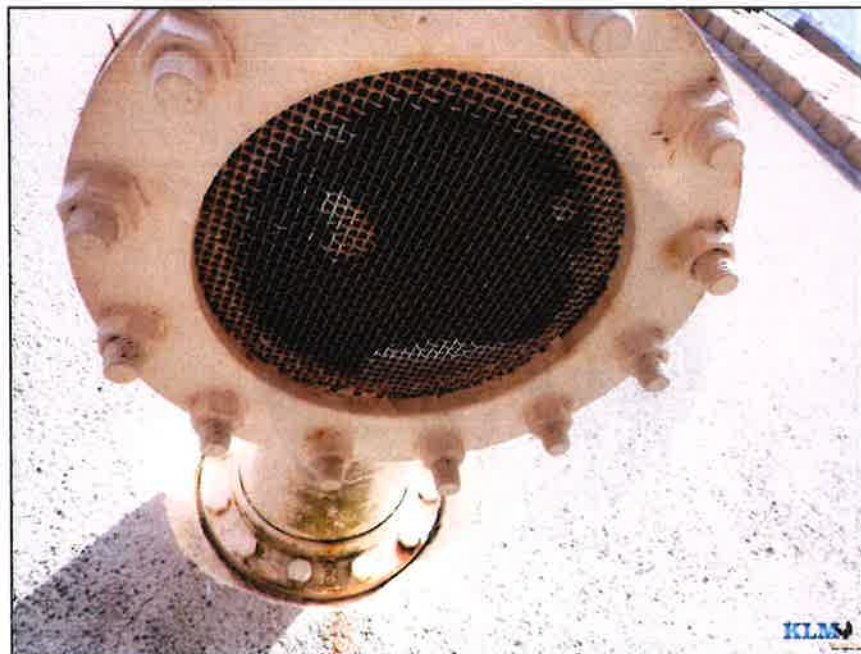
Photo No. 20 Condition of overflow pipe screen
