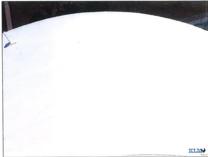
Photo No. 15 Roof coating conditions
