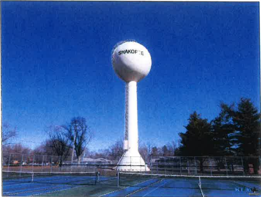
Photo No. 1 Overall view of the tower
