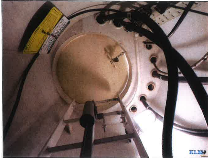
Photo No. 9 Top of drywell tube (looking up)
