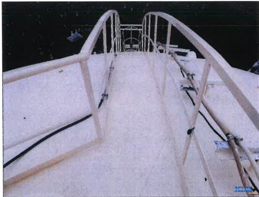
Photo No. 12 Roof handrail and access
