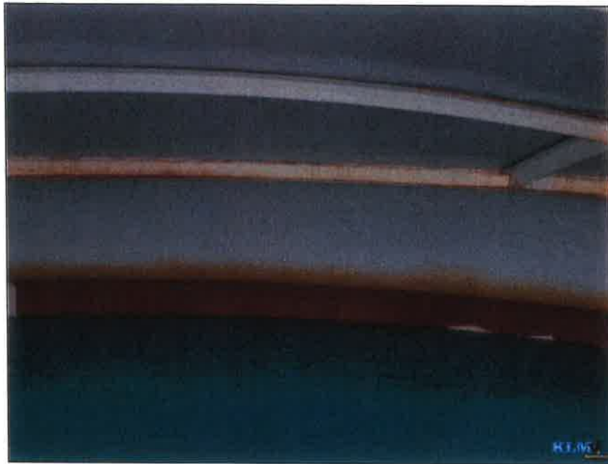
Photo No. 5 Condition of roof and upper shell
