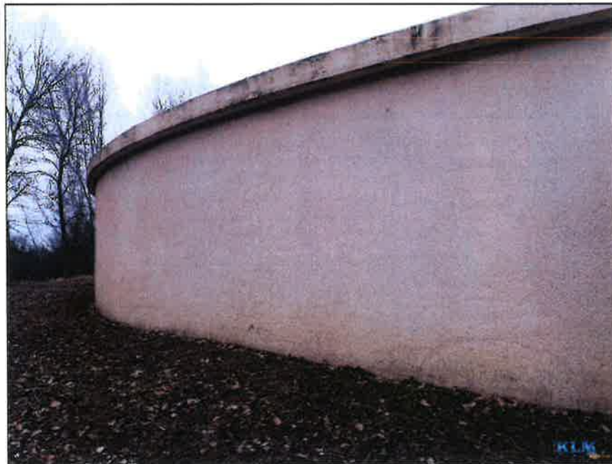
Photo No. 12 Typical wall condition
