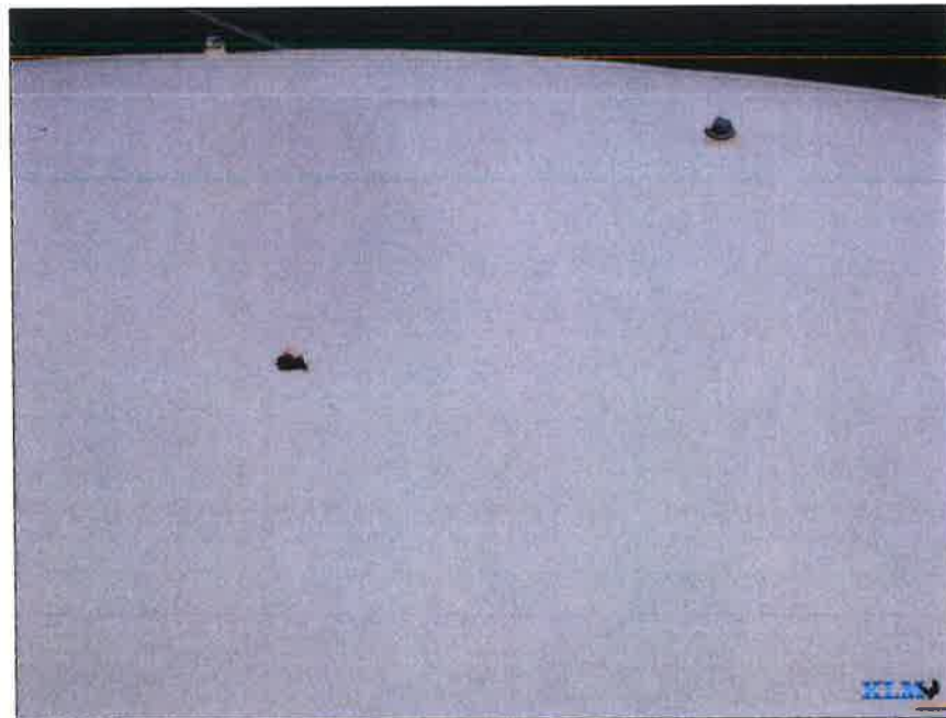
Photo No. 8 Coating conditions on roof
