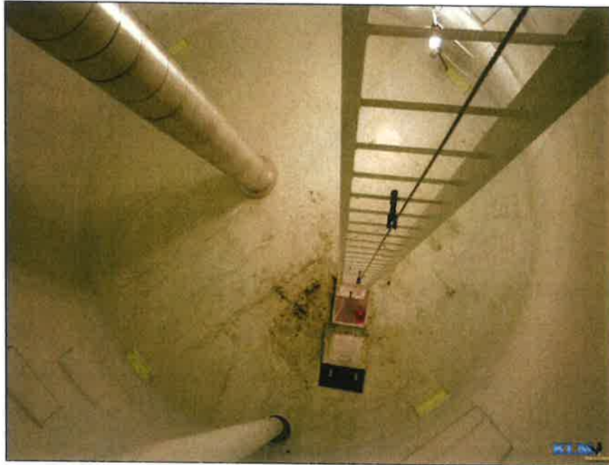
Photo No. 33 View of bottom landing
