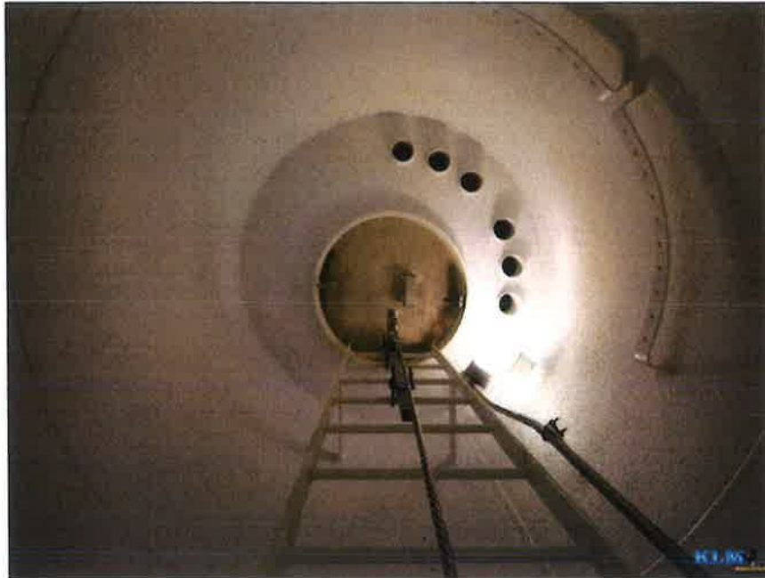
Photo No. 23 Top of drywell tube (looking up)
