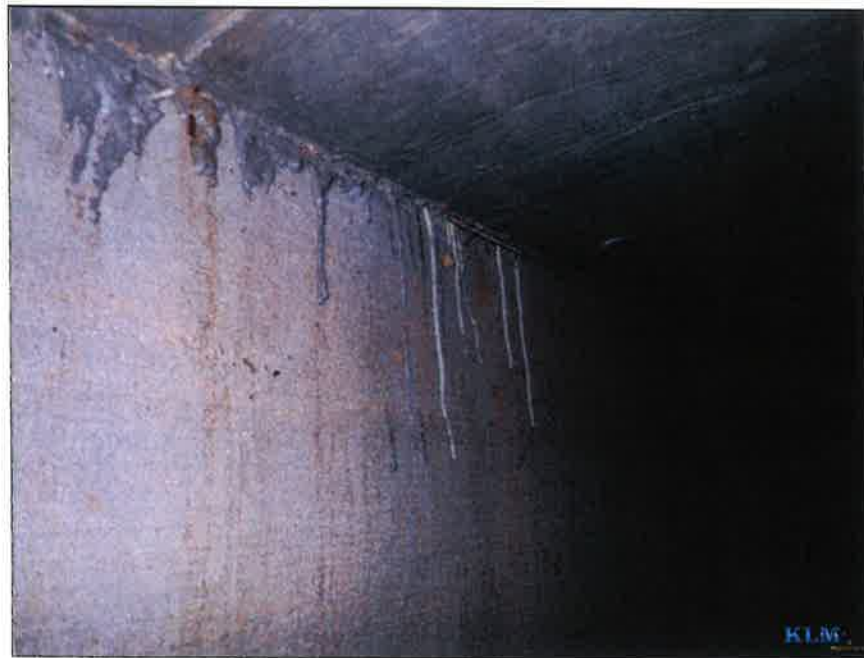
Photo No. 6 Condition of wall
