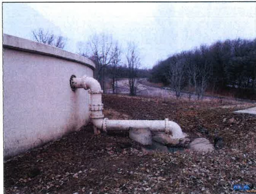
Photo No. 16 Overflow pipe and catch basin
