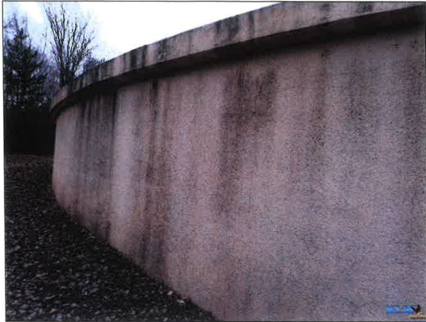
Photo No. 13 Typical wall condition
