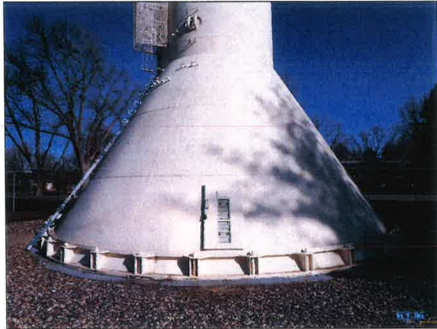
Photo No. 19 Base cone with view of door
