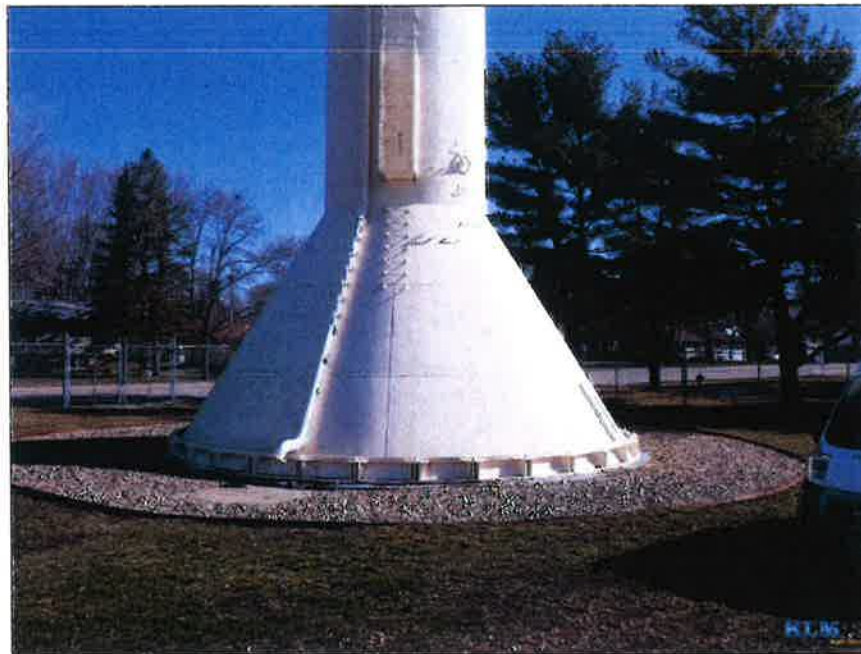
Photo No. 20 Base cone with view of overflow pipe
