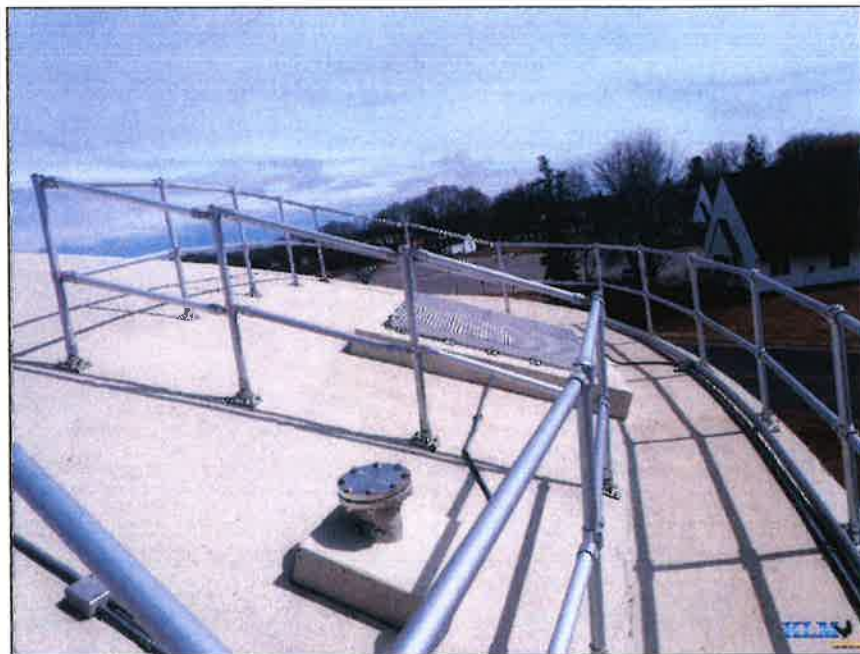
Photo No. 12 Roof handrailing
