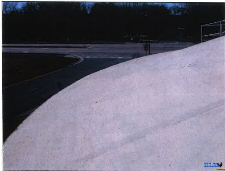
Photo No. 10 Typical condition of roof coating
