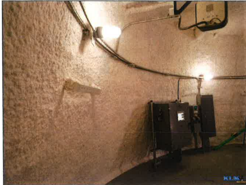
Photo No. 35 Base cone conditions
