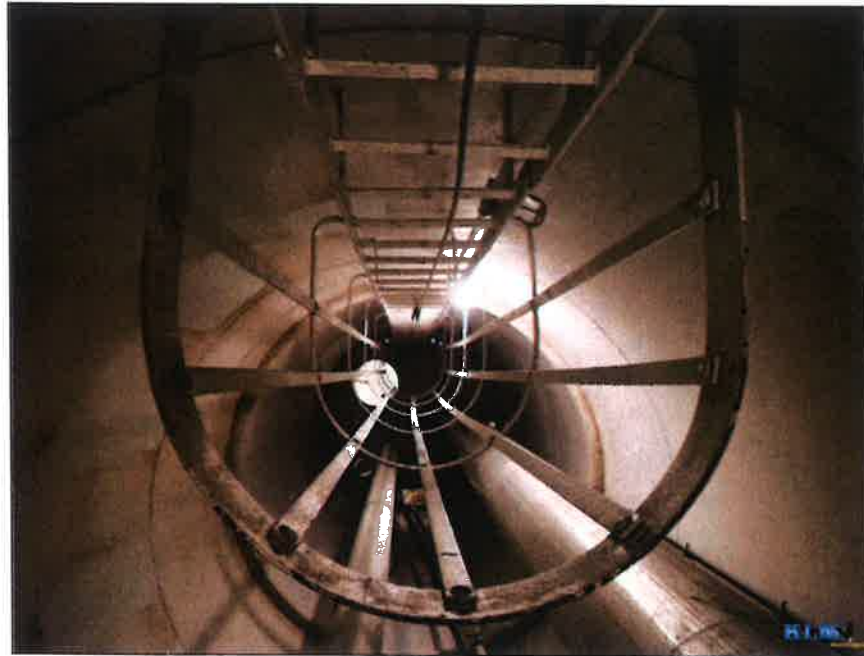
Photo No. 14 Overall conditions in riser
