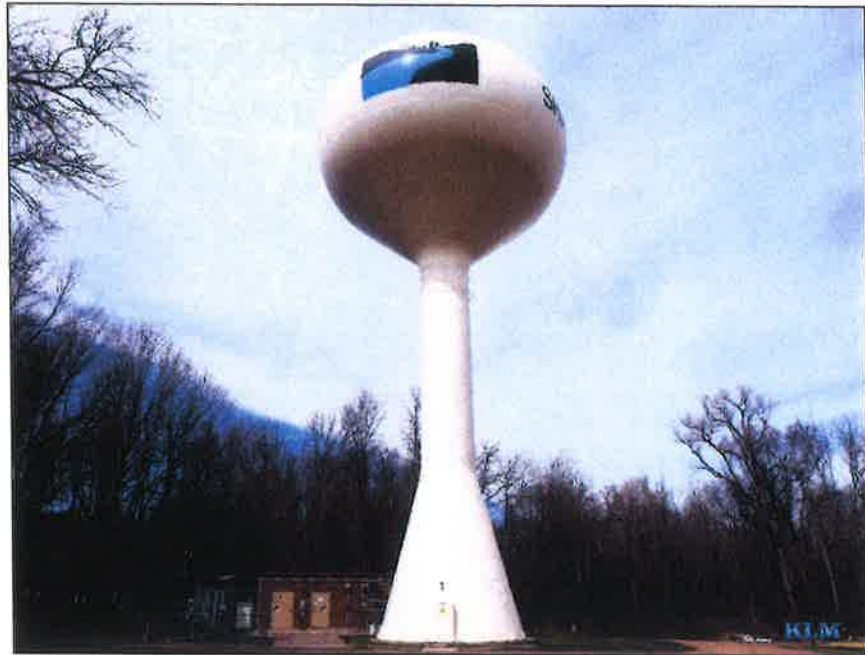
Photo No. 1 Overall view of tower
