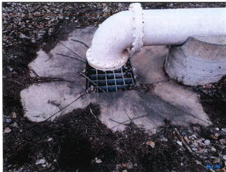
Photo No. 16 Condition of overflow pipe and grating
