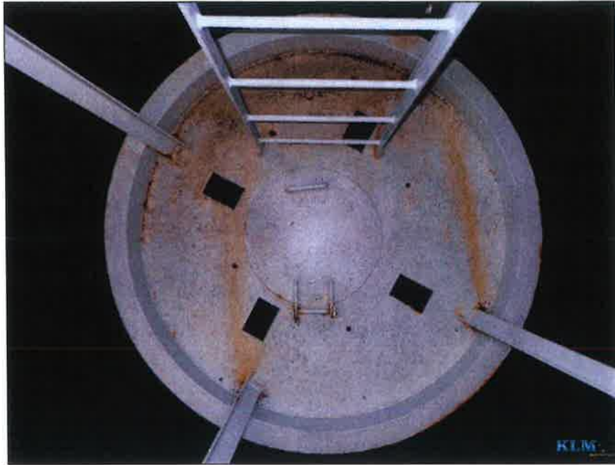
Photo No. 7 Inspection platform
