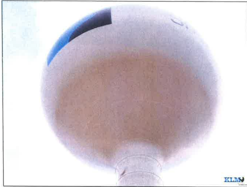
Photo No. 21 Overall condition of water compartment
