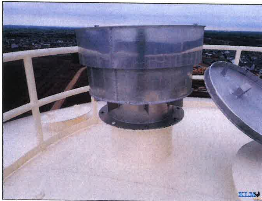
Photo No. 38 Finial vent
