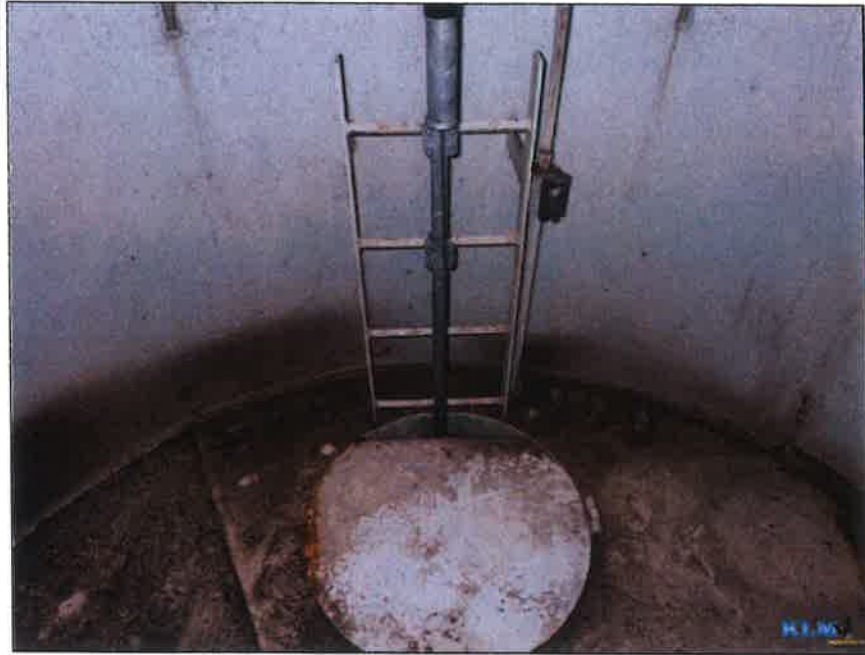
Photo No. 13 Conditions of top landing
