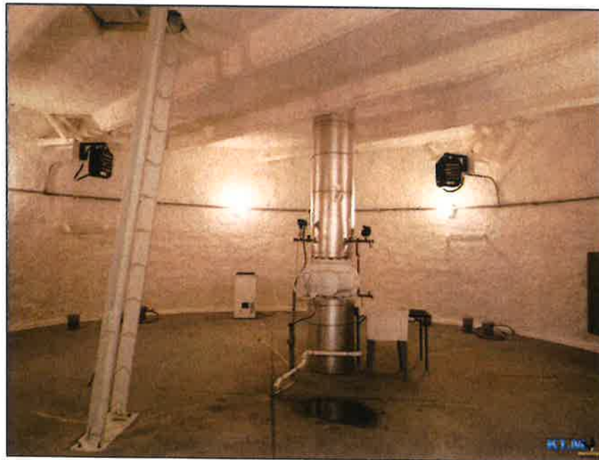
Photo No. 34 Base cone conditions
