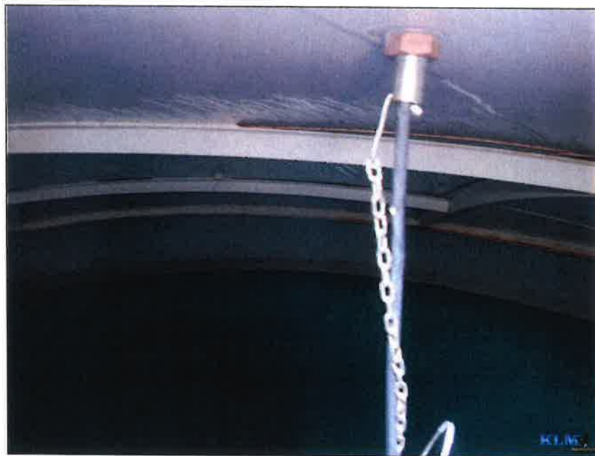
Photo No. 2 Interior roof conditions
