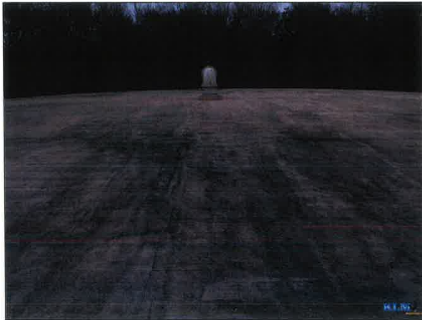
Photo No. 11 Condition of roof coating
