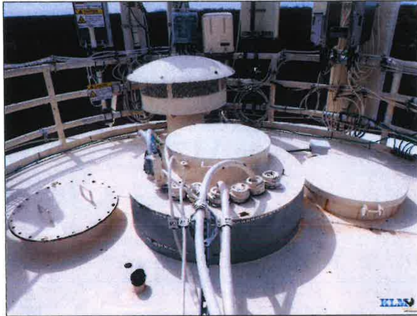
Photo No. 19 Overall conditions on roof Note: finial vent
