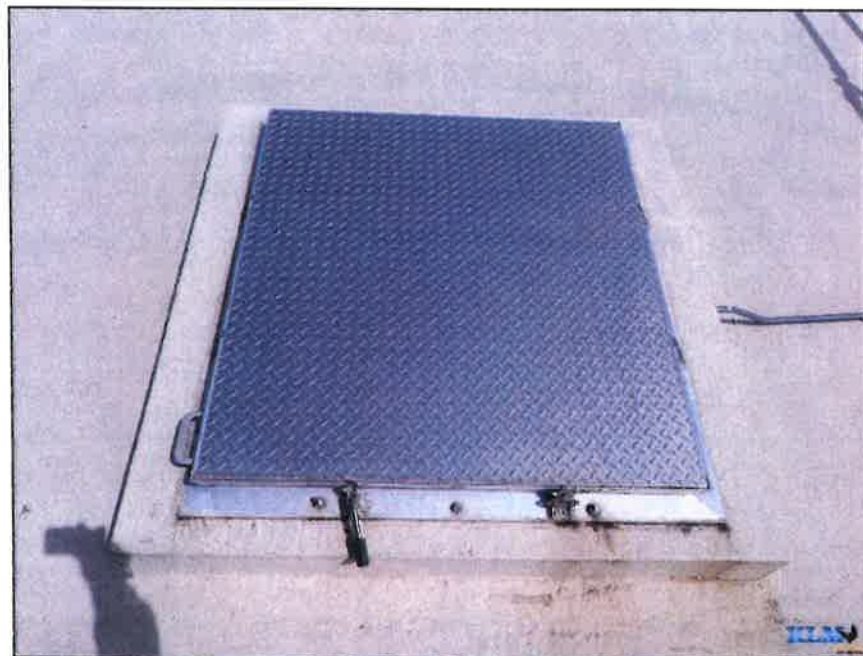
Photo No. 14 Roof hatch and interior ladder
