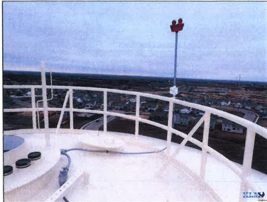
Photo No. 39 Roof conditions Aviation light visible
