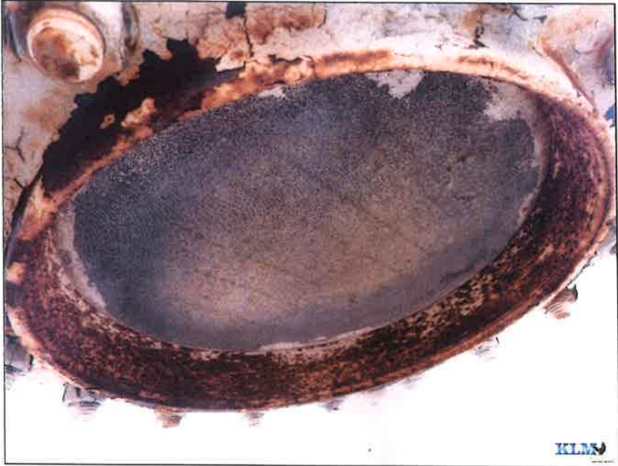
Photo No. 17 Condition of overflow pipe screen
