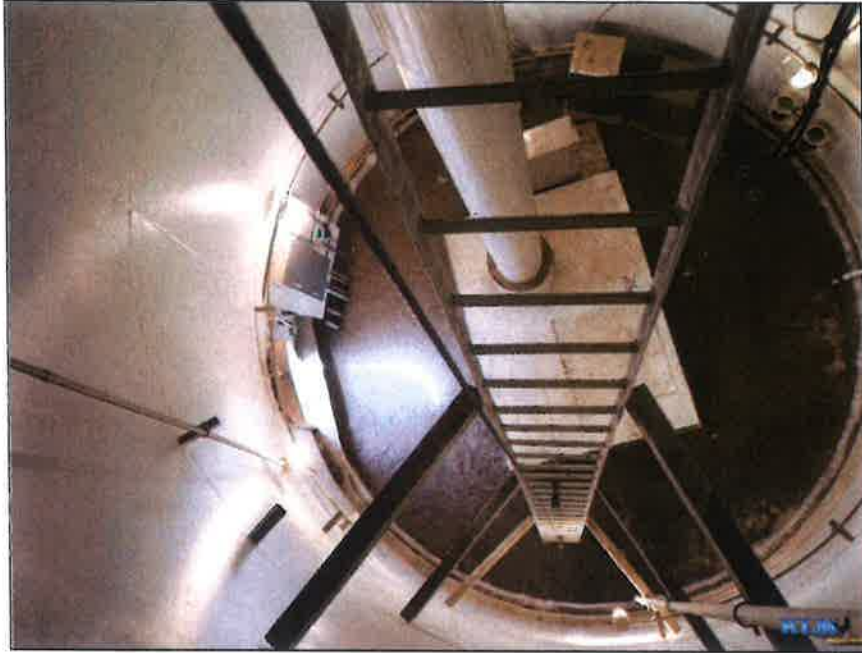
Photo No. 17 Overall conditions in base of tank
