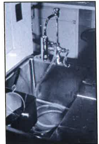
FIGURE 17. Atmospheric vacuum breaker in plumbing supply system.
