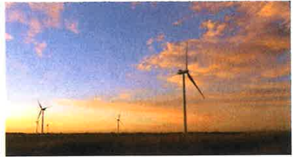
OAK GLEN WIND FARM STEELE COUNTY, MN 44 MW, WIND
