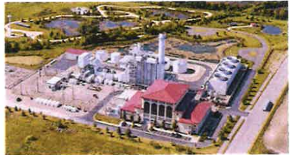
FARIBAULT ENERGY PARK FARIBAULT, MN 300 MW, NATURAL GAS
