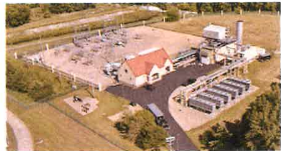
MINNESOTA RIVER STATION CHASKA, MN 49 MW, NATURAL GAS
